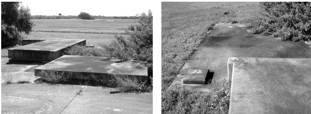
Figure 60. Removable concrete covers over Silo 32B R&D equipment room (left foreground) and subterranean staircase (left background; right foreground); concrete roof with corner exhaust vent of transformer vault (right background) (ERDC-CERL 2007).
