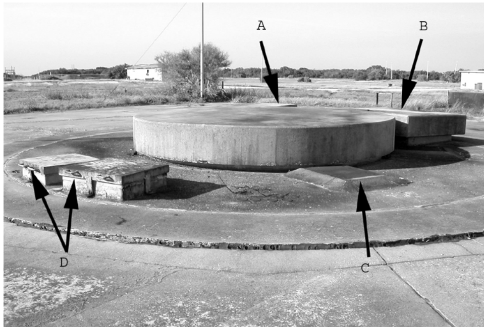
Figure 59. Silo 31B showing (A) guidance alignment notch, (B) personnel and equipment access hatch, (C) T-E jack point, and (D) junction-box openings (ERDC-CERL 2007).
