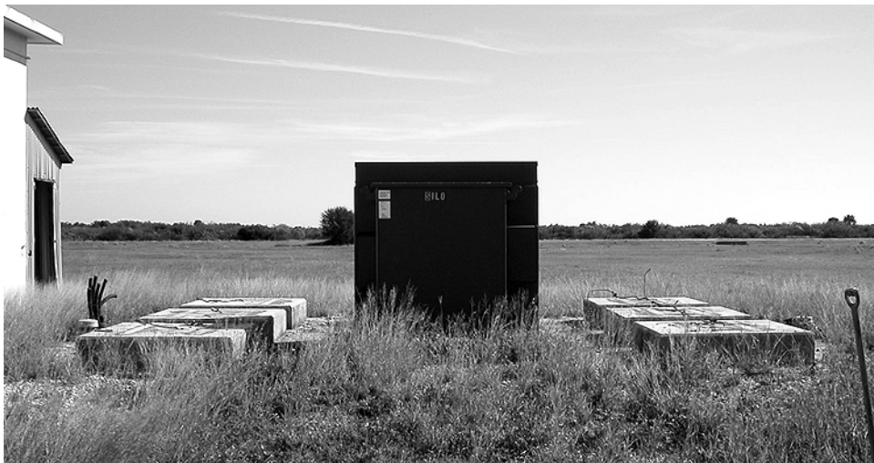
Figure 67. Launch support building transformer vault (ERDC-CERL 2007).
