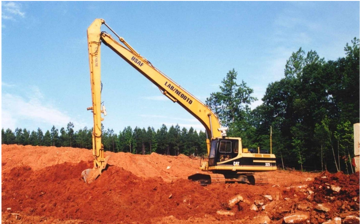
Figure 2: Remote Controlled Caterpillar 325L Excavator
