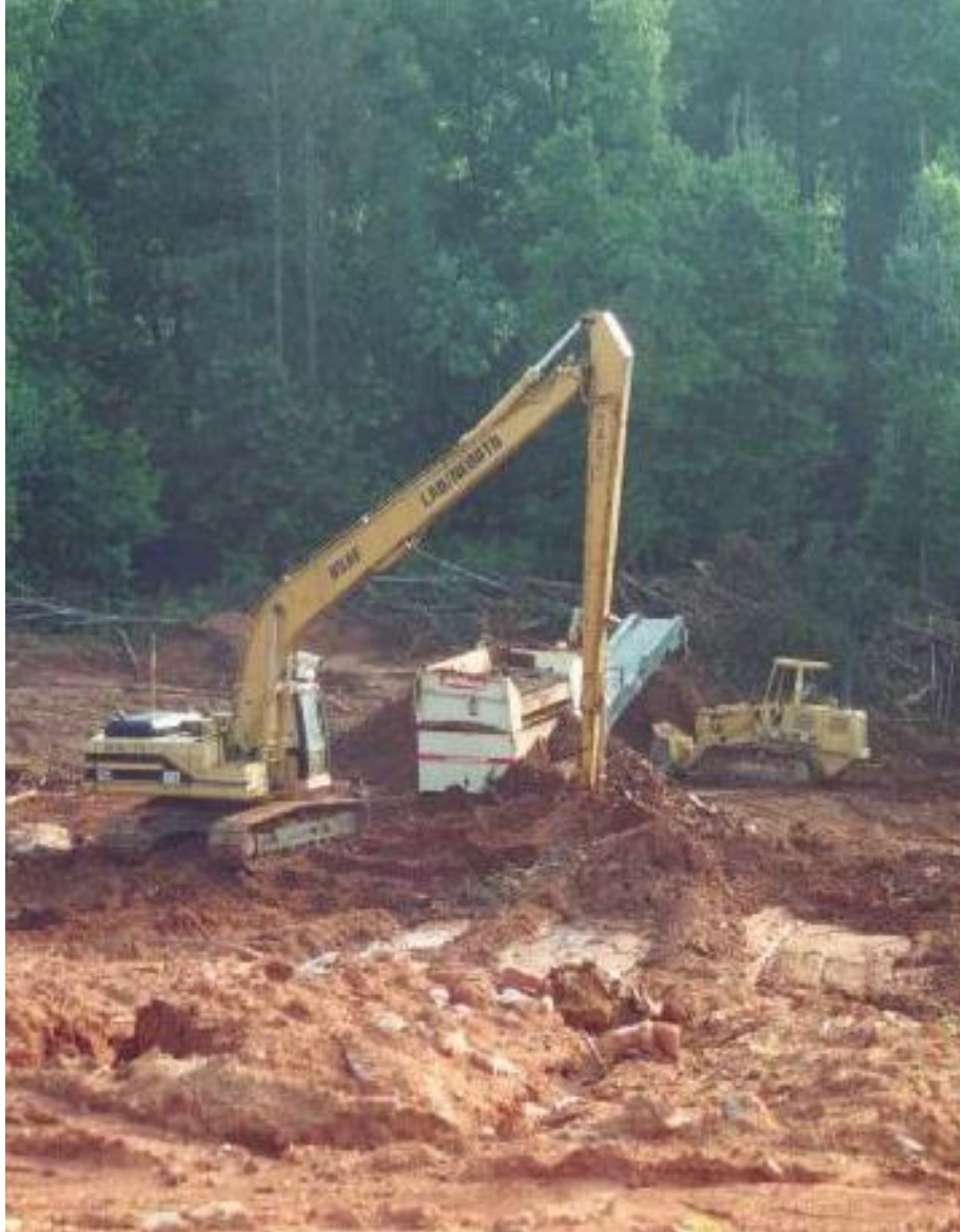
Figure 6: Excavator and Sifter/Shaker Site Location
