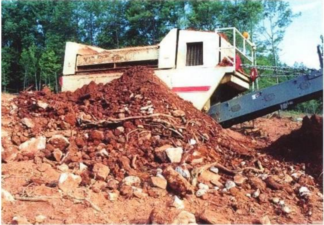
Figure 4: Self-Propelled Nordberg ST170 Sifter/Shaker On-Site
