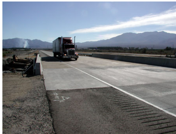
Figure 12. The Kings Stormwater Channel Bridge deck in California achieves composite bending action with carbon composite shell girders filled with lightweight concrete.
