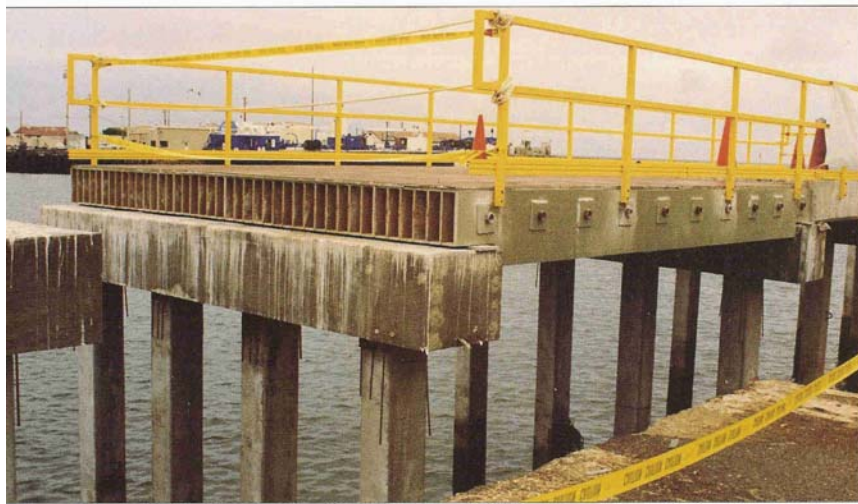
Figure 22: NFESC's Advanced Waterfront Technology Test Site all-composite deck.
