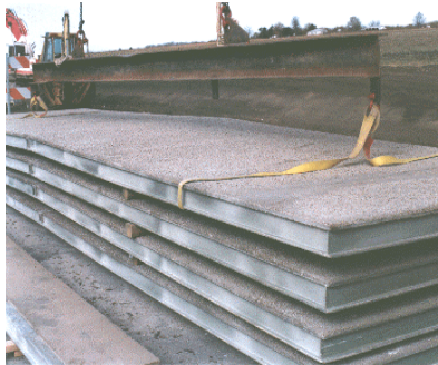
Figure 5. FRP composite bridge deck panels for installation on Kansas State Highway 126 west of Pittsburg, Kansas. Panels manufactured by Kansas Structural Composites Inc.
