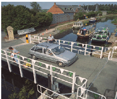
Figure 7. The Bonds Mill Lift Bridge in Stonehouse, England was one of the first FRP bridges built for vehicular traffic (1994).
