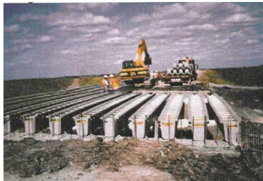
Figure 24. U-shaped FRP beams for TxDOT San Patricio County bridge.
