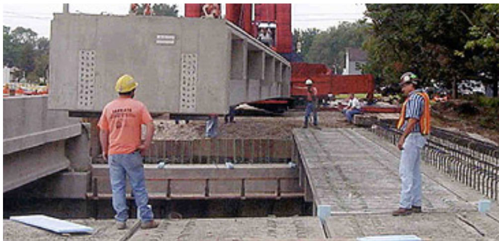
Figure 3. Installation of CFRP reinforced concrete sections on the Bridge Street Bridge.
