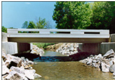
Figure 6. Modular FRP bridge in West Virginia manufactured by Creative Pultrusions.
