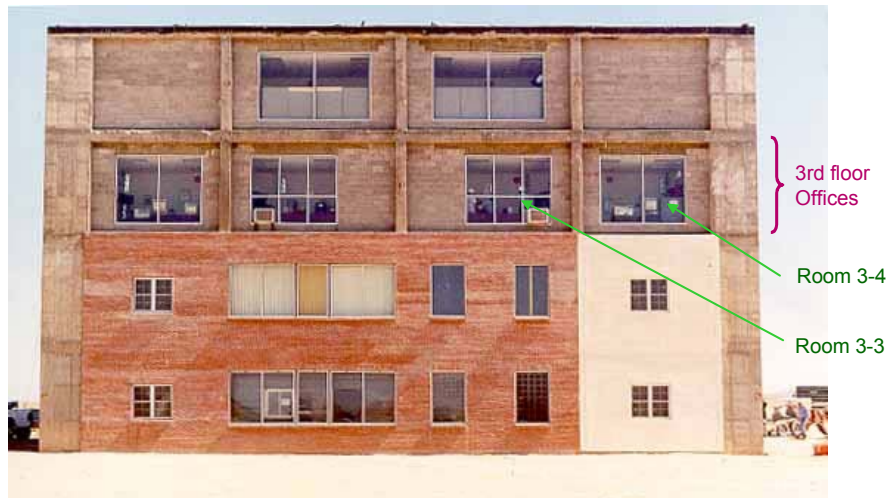
Figure 2. Front face elevation of simulated office building.
