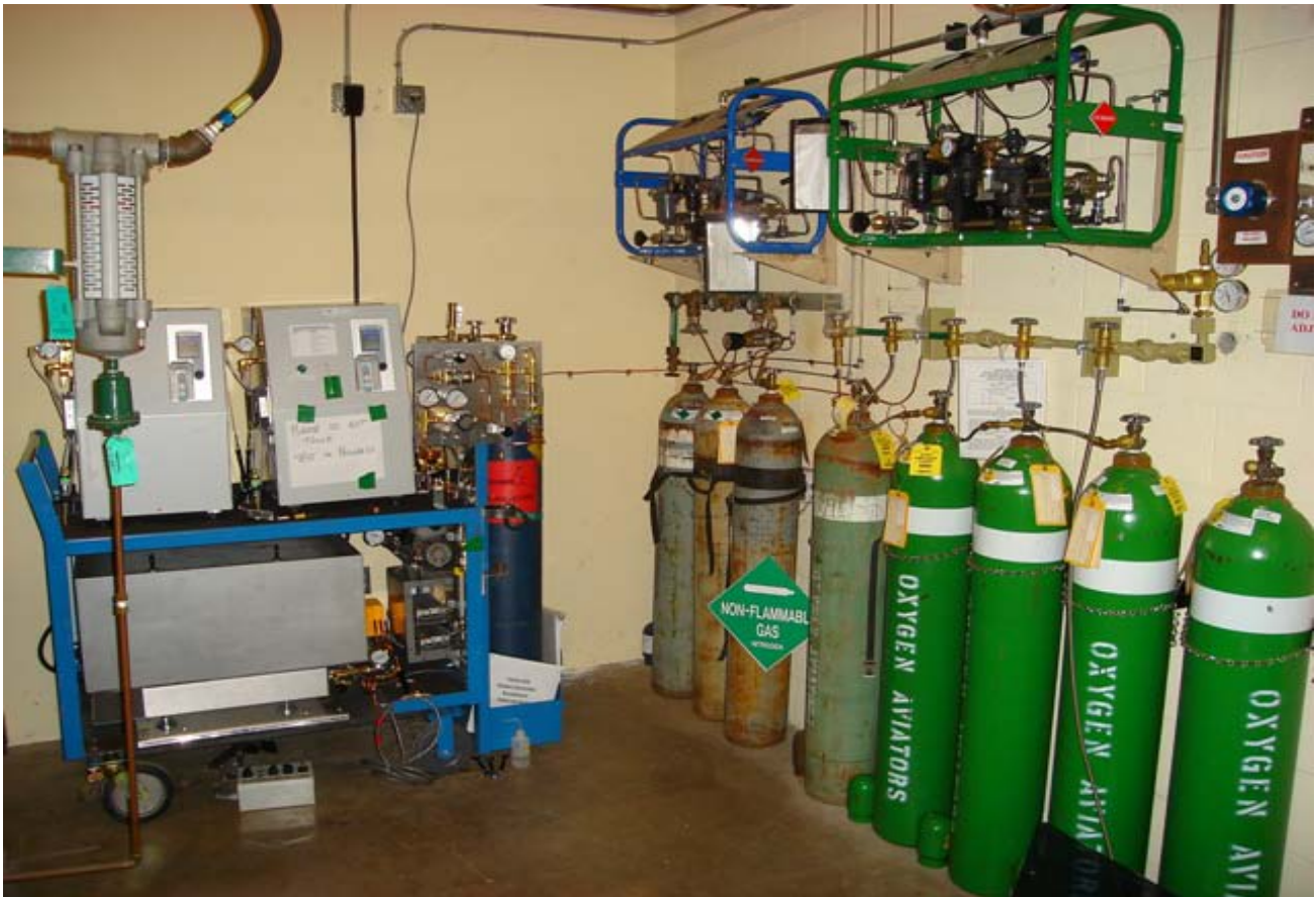
Photograph #2. SEOS breadboard shown with facility high pressure oxygen supply system.
