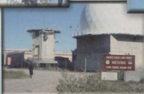
Kotzebue Long Range Radar Site, Kotzebue, AK Photos by Chris Elmer.
