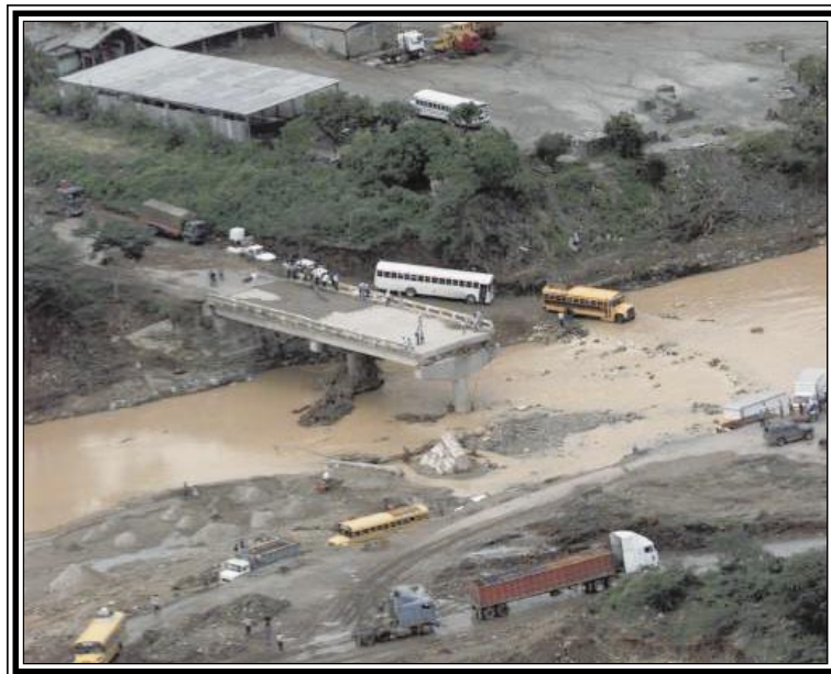
The floods following Hurricane Mitch washed out many roads and knocked down bridges like this one near Yoro, Honduras DoD Photo by: TSGT Thomas Cook, Soto Cano Air Base
