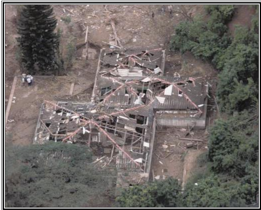
Aerial view of some of the destruction caused by Hurricane Mitch in Honduras DoD Photo: TSGT Thomas Cook, Soto Cano Air Base
