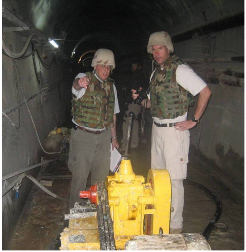
Site Photo 43. SIGIR inspector pointing out an active grout pump placing grout into a hole
