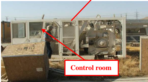
Site Photo 14. Concrete batch-mixing plant control room
