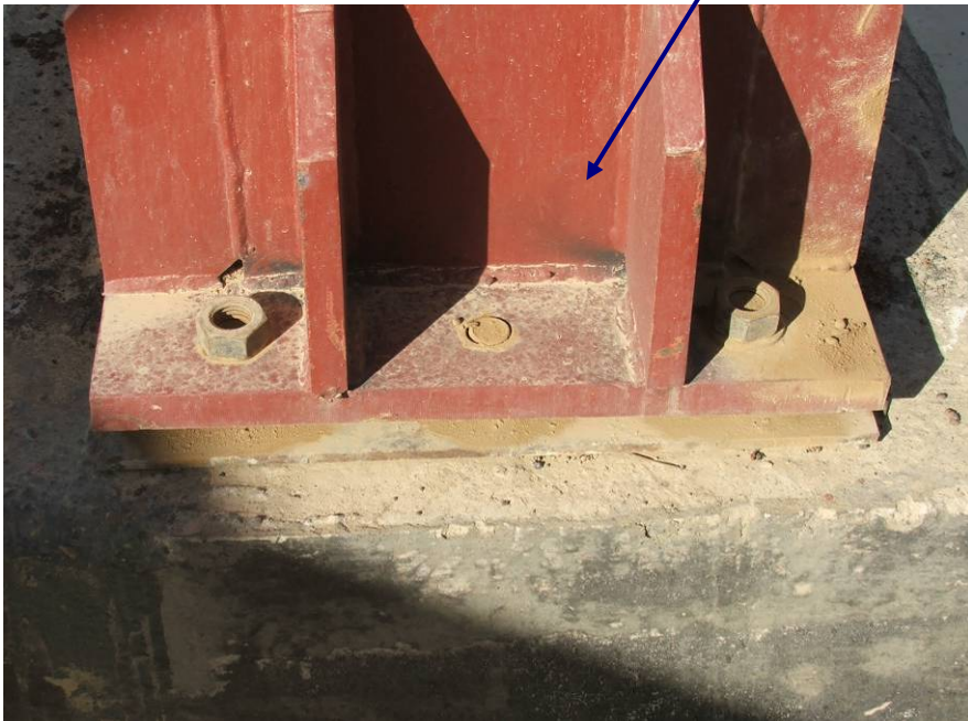
Site Photos 18 and 19. Close-up view of foundation bolts for the stationary silos
