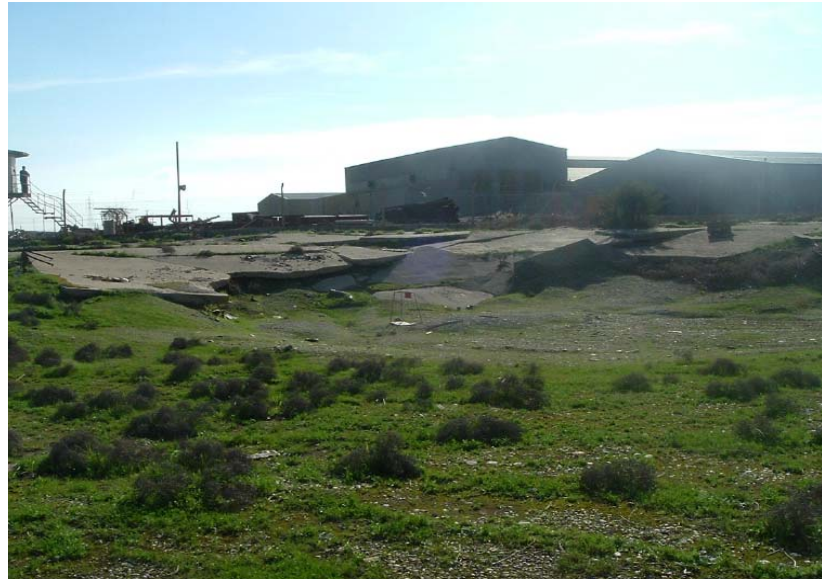
Site Photo 9. Sinkhole beneath a concrete-paved area (Photo courtesy of the USACE)
