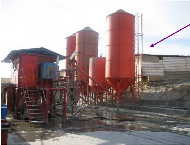
Site Photo 10. Existing 20- \text{m}^3/\text{hour} grout-mixing plant (Photo courtesy of the Iraq Transition Assistance Office (ITAO))
