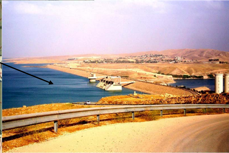
Site Photo 1. Mosul Dam (Photo courtesy of the USACE)
