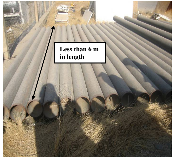
Site Photo 26. Pipes delivered by the contractor
