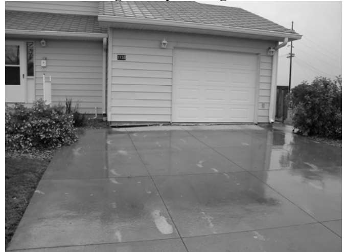
Figure 1. Damaged military housing in the Minuteman Village family housing area.
