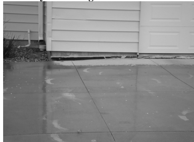
Figure 2. House separated from foundation caused by excessive ground movement.
