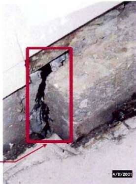
Foundation cracking and floor separating from foundation
