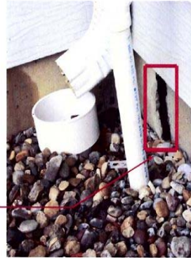
Foundation crack
