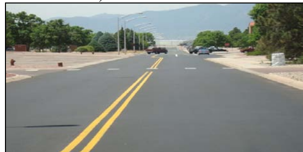
Figure 2. Lighting, gas and pavement repairs on Otis Street, Peterson Air Force Base
