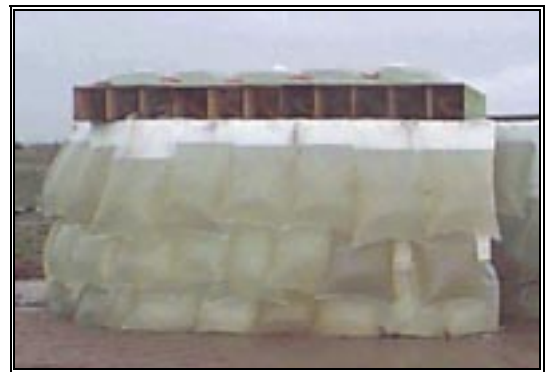
Poldine Bomb Shelter (walls and roof).
