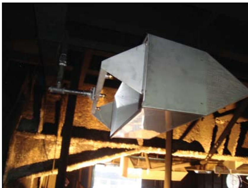
FIGURE 1 HofFoam HG-25 generator mounted in the overhead grid system.
