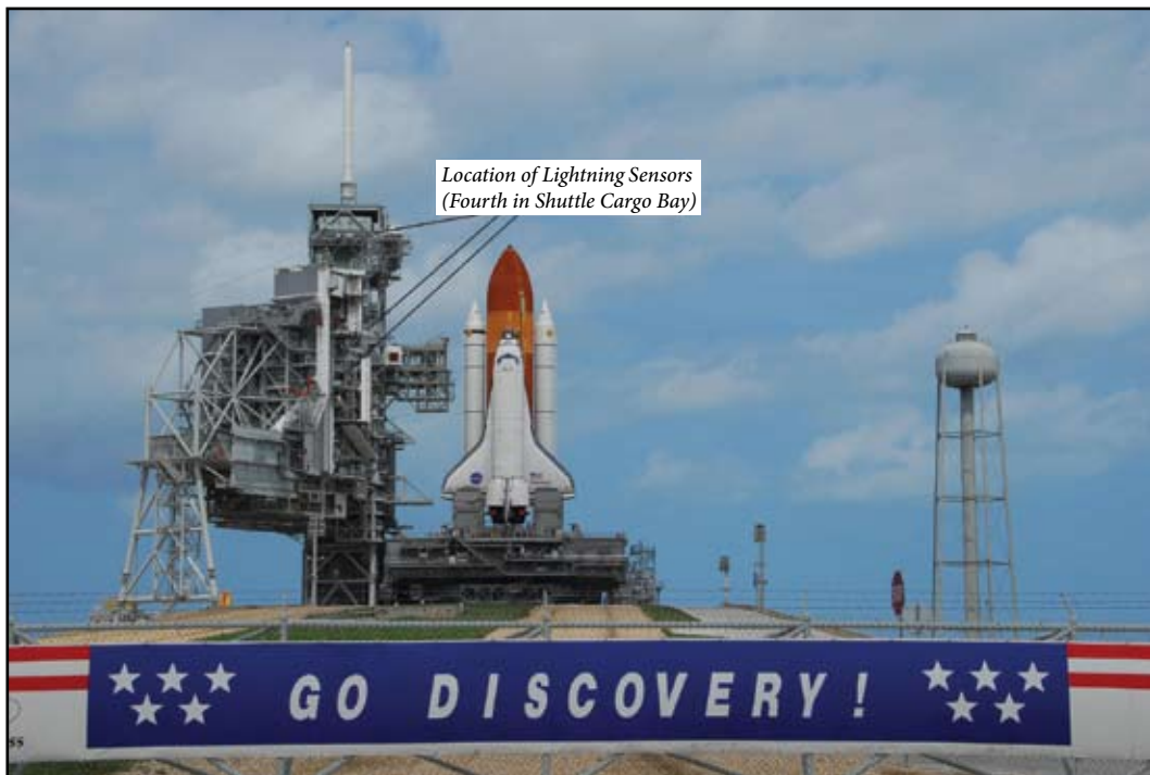
FIGURE 7 GLMS placement on the space shuttle Discovery launch pad.
