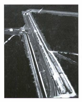
Completed in 1967, Dahlgren's half-mile-long conical shock tube allowed DASA and NWL scientists to simulate 20-kiloton nuclear explosions without using radioactive materials. (Dahlgren Historic Photograph Collection)
