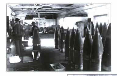
In 1945, inert projectiles are being prepared in the Shell House for testing.
