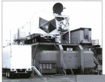
From 1987 through 1995, ship defense anti-air warfare radar systems installed at Dahlgren's Land Based Sensor Test Site supported a variety of programs to improve sensor performance for the detection of low altitude, low radar cross-section, fast incoming missiles. (Dahlgren Historic Photograph Collection)
