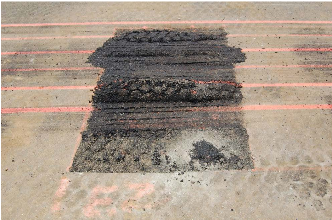
Figure 31. Failure in repair 1 EZ-Street.
