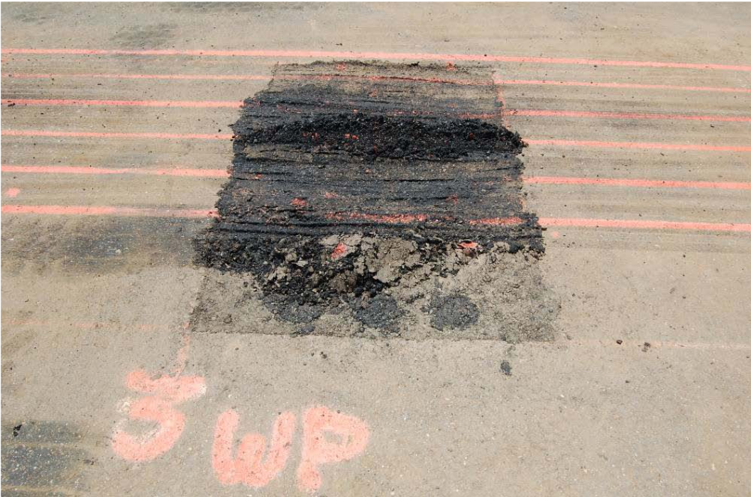
Figure 33. Failure in repair 3 Wespro.
