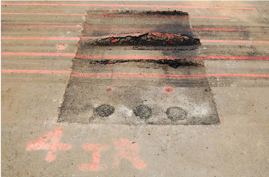
Figure 34. Failure in repair 4 Instant Road Repair.
