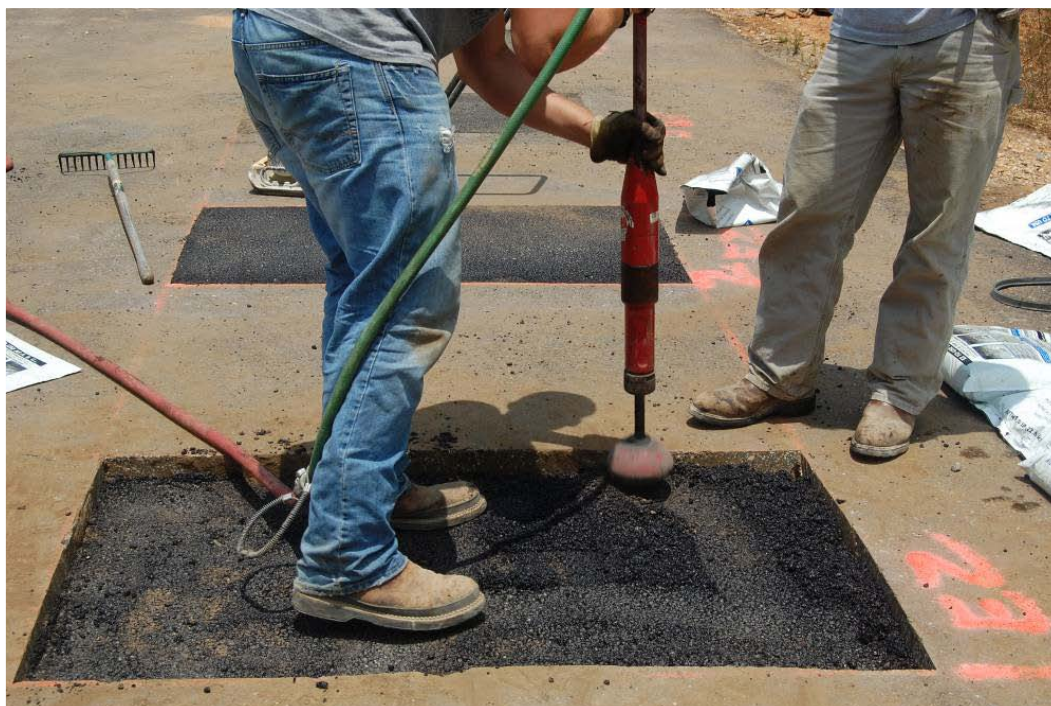
Figure 23. Pneumatic tamping compactor with a 5-in. circular head.
