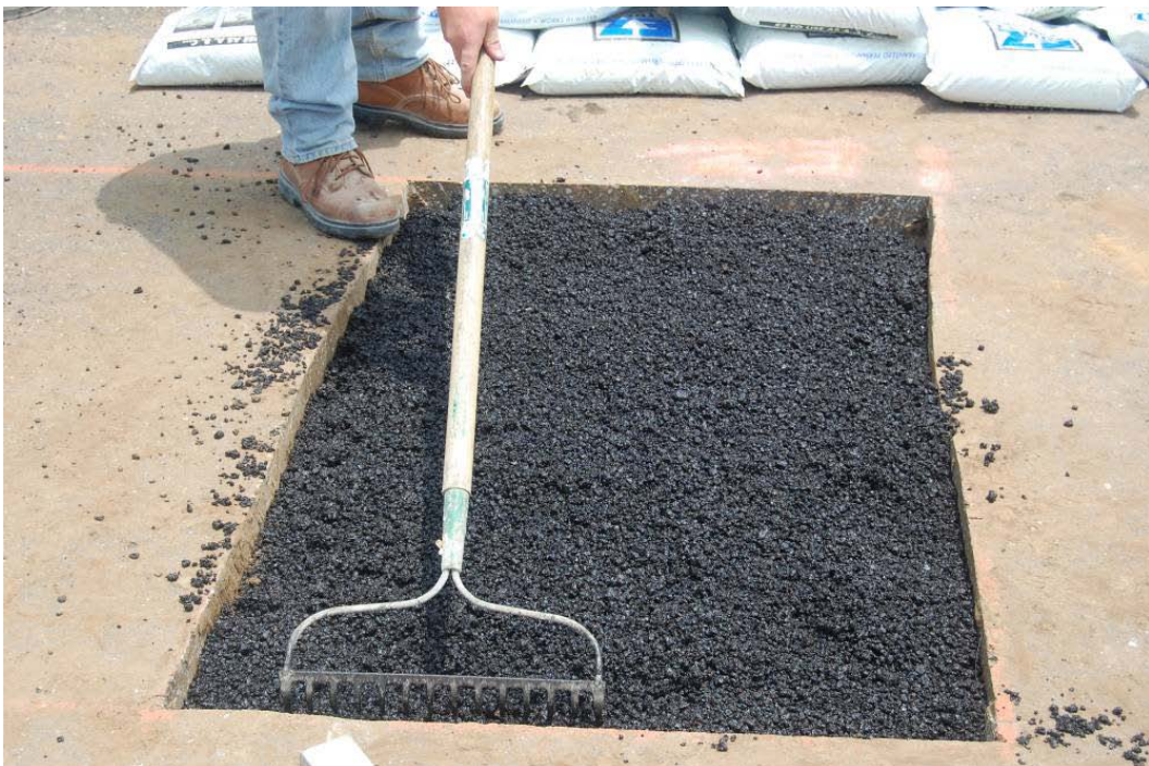
Figure 22. Spreading of the material.
