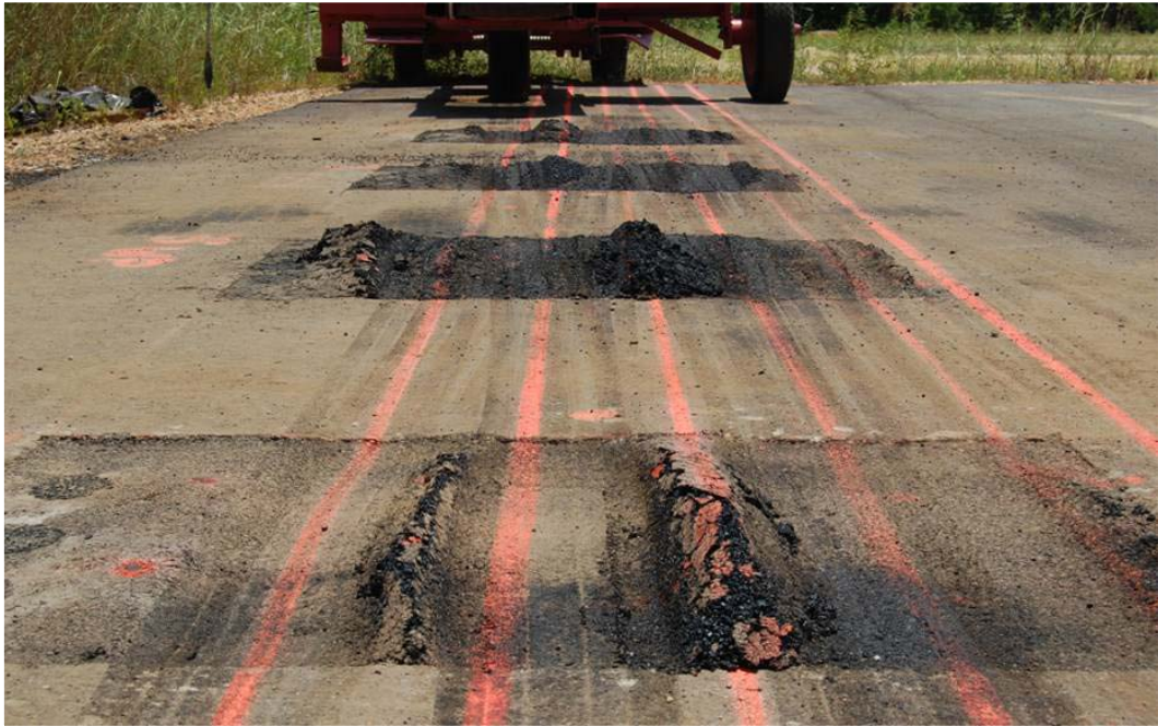
Figure 35. Overall photo of the repairs after 16 passes.
