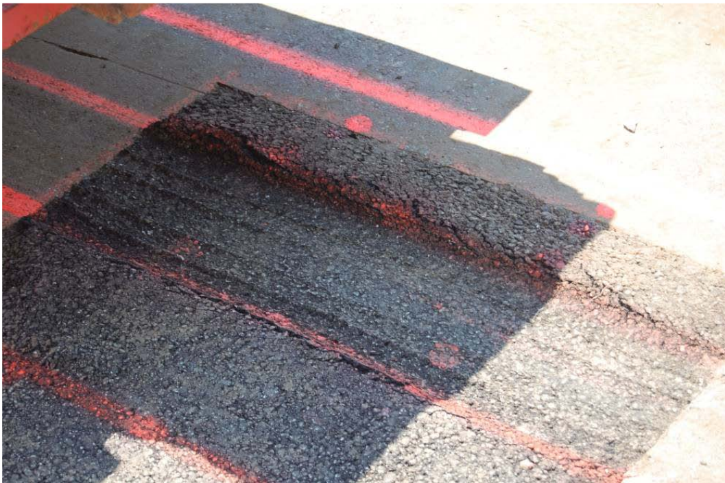
Figure 30. Deformation after the third pass over Instant Road Repair.
