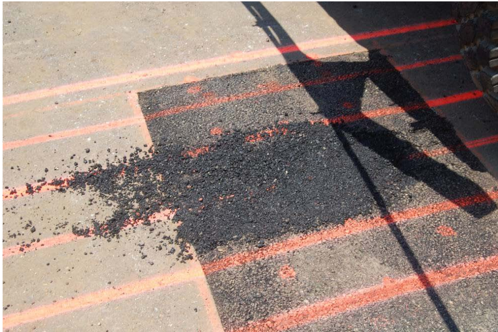
Figure 29. Damage in the EZ-Street Hybrid product.
