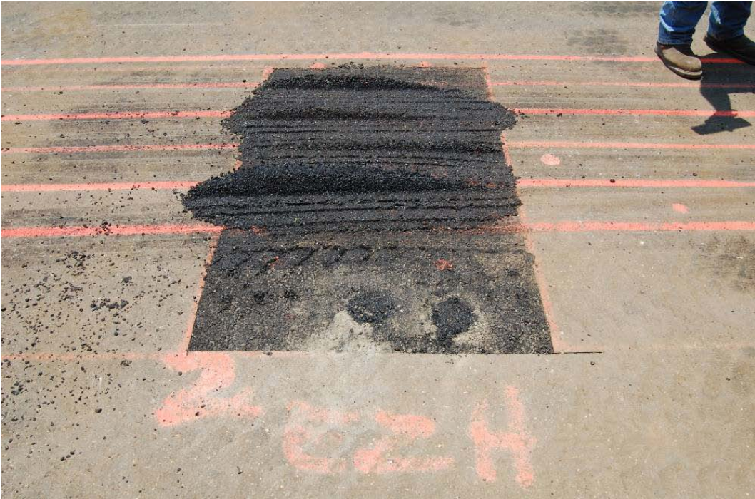
Figure 32. Failure in repair 2 EZ-Street Hybrid.
