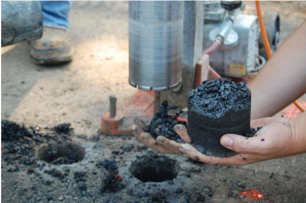
Figure 25. Core sample falling apart due to high air voids in the mix.
