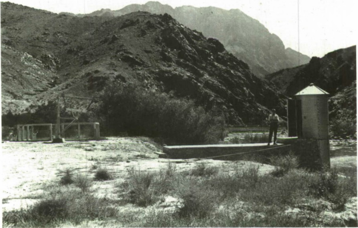
Figure 3.--One of 63 new streamgaging and weather stations built by Surface Water Research project. Automatic water stage recorders are installed in structure on right; weather observation instruments will be installed in enclosure on left.
