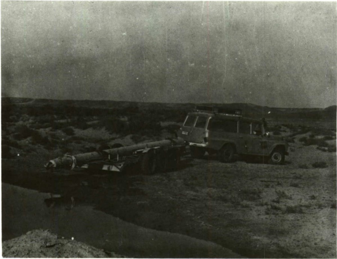
Figure 8.--Transporting specially-designed telescoping column support across Dasht-i-Margo desert. The transport length of 27 feet extended to 45 feet when erected.
