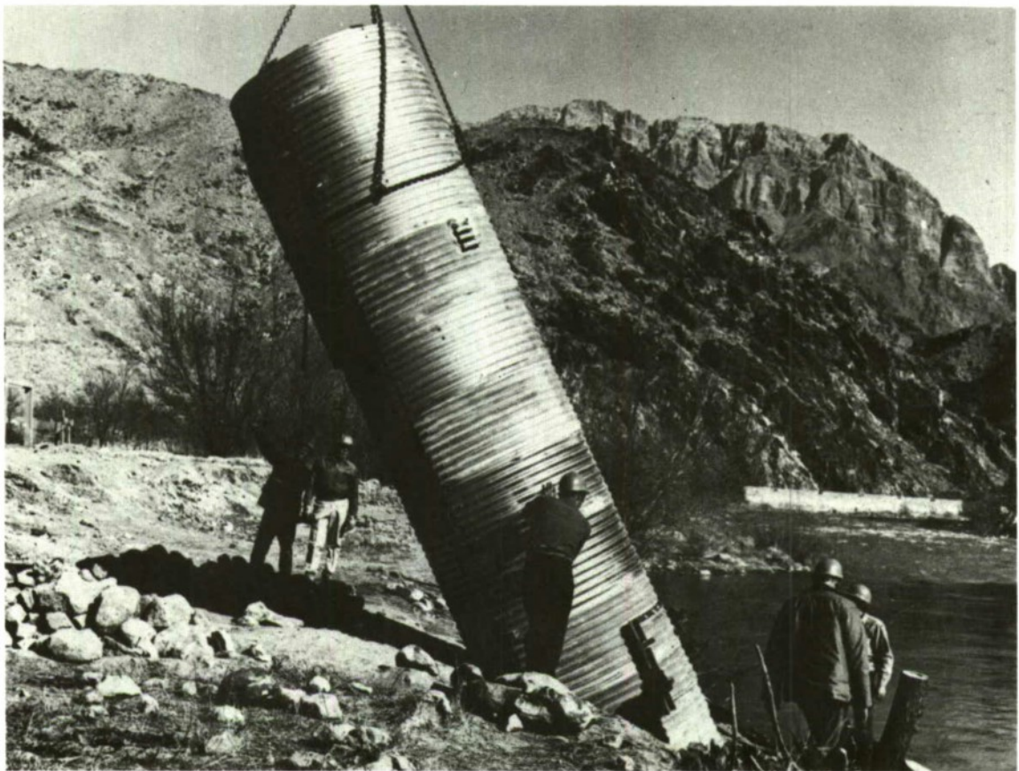
Figure 4.--Afghan counterparts learning stilling well installation from A. O. Westfall.
