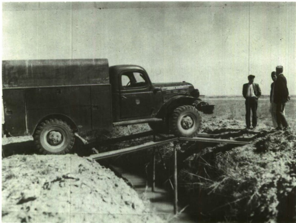
Figure 6.--Portable bridge over canal in Chakansur area designed and built by I. A. Heckmiller, Hydrologic Advisor.
