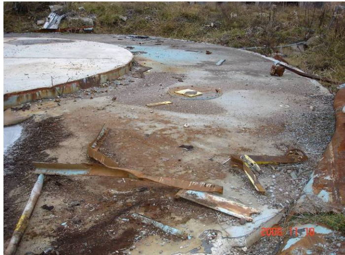
Figure 271. Foundation of fuel oil tank.
