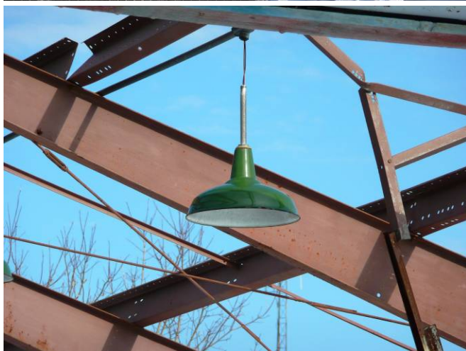
Figure 214. Exterior of light fixture and structure of steel framed storage building.
