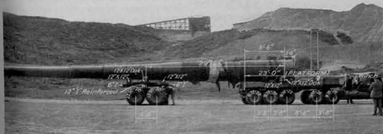
160 Tons—the heaviest load ever carried by pneumatic tires.
