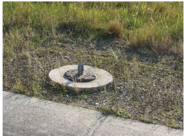
Missing Runway Lights at NAS/JRB New Orleans
