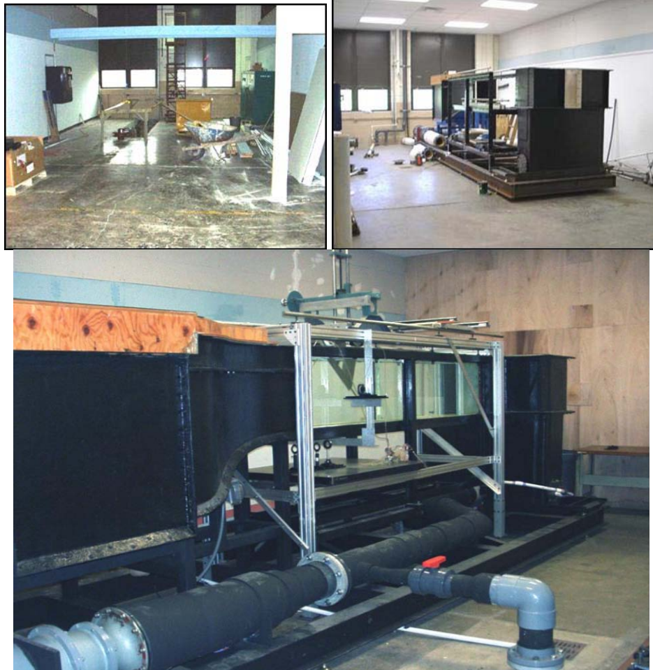
Figure 8. HFWT installation history: site preparation, including excavation for sewer drain (top left); mockup of main components on support frame, without connecting plumbing and test section glass walls (top right), and tunnel operational (above).
