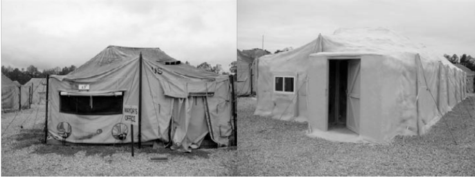
Figure 3. Tent Before and After Application of Foam Insulation
