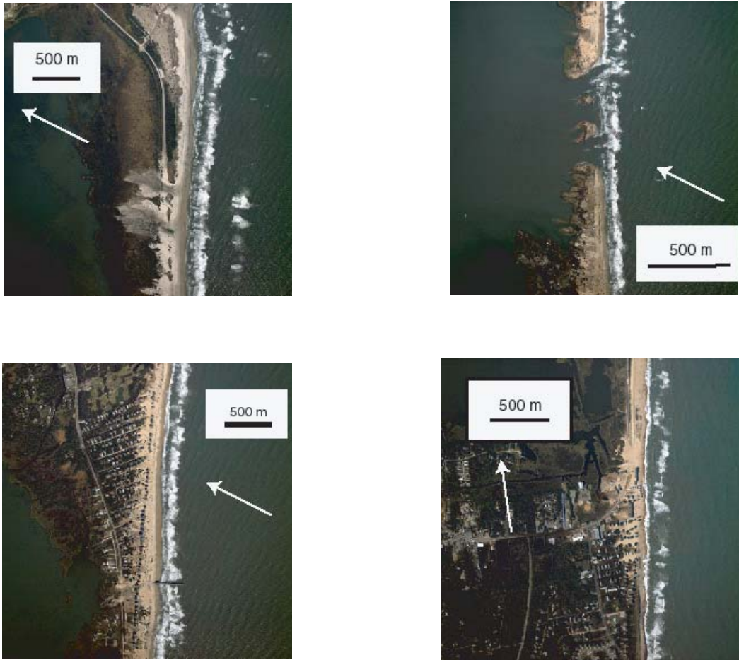
Figure 13. Aerial photographs taken after Hurricane Isabel on the Outer Banks (see Fig. 1B for locations). (A) Ocracoke Island; (B), Cape Hatteras National Seashore; (C) Frisco; and (D) Buxton. The photographs are oriented with Pamlico Sound to the left. The arrows indicate north.
