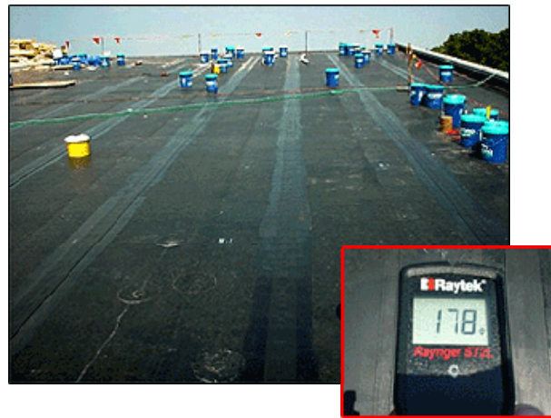
Figure 4. Roof before treatment; Thermometer reads 178 °F.
