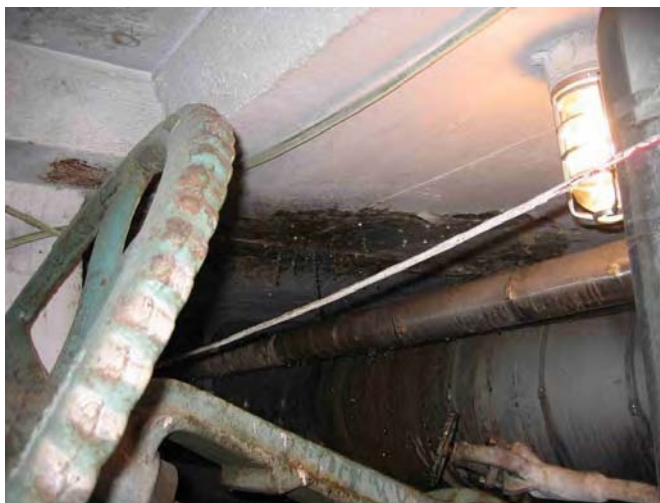
Figure 15. Leak in a condensate line.
