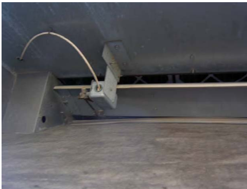
Figure 32. Fixed outside air damper.
