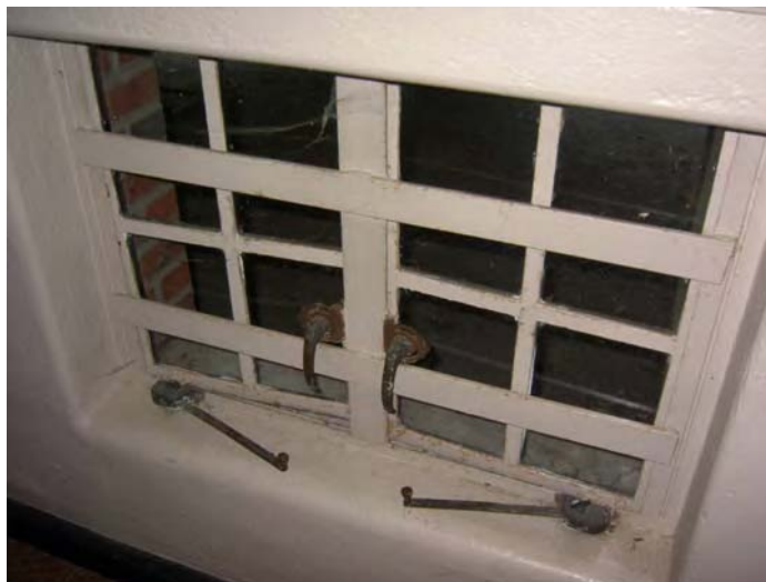
Figure 7. Basement windows of Building 685 (which do not close ).
