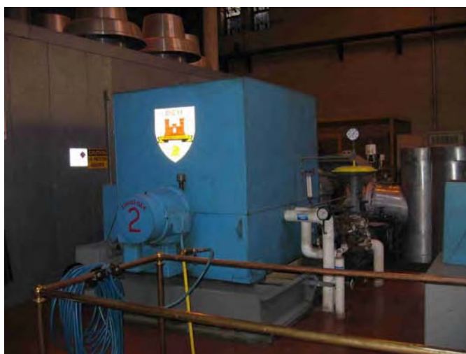
Figure 21. Backpressure steam turbine #2 in CEP 604.
