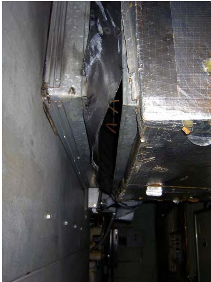
Figure 11. Large gap in the supply duct, Building 622, Library.
