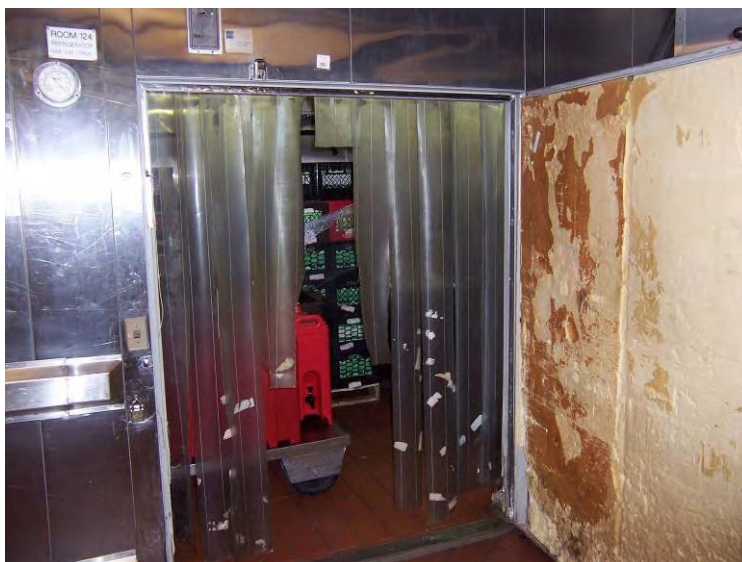
Figure 34. Damaged door to refrigerated room, i.e., no inside metal covering exposed insulation (note opening in plastic strips).
