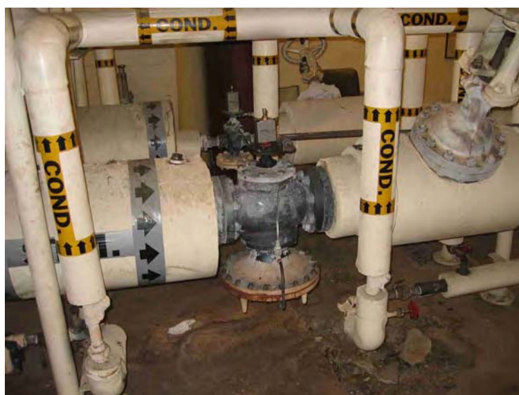
Figure 20. Pressure reducing valves in Building 745A (Mess Hall).
