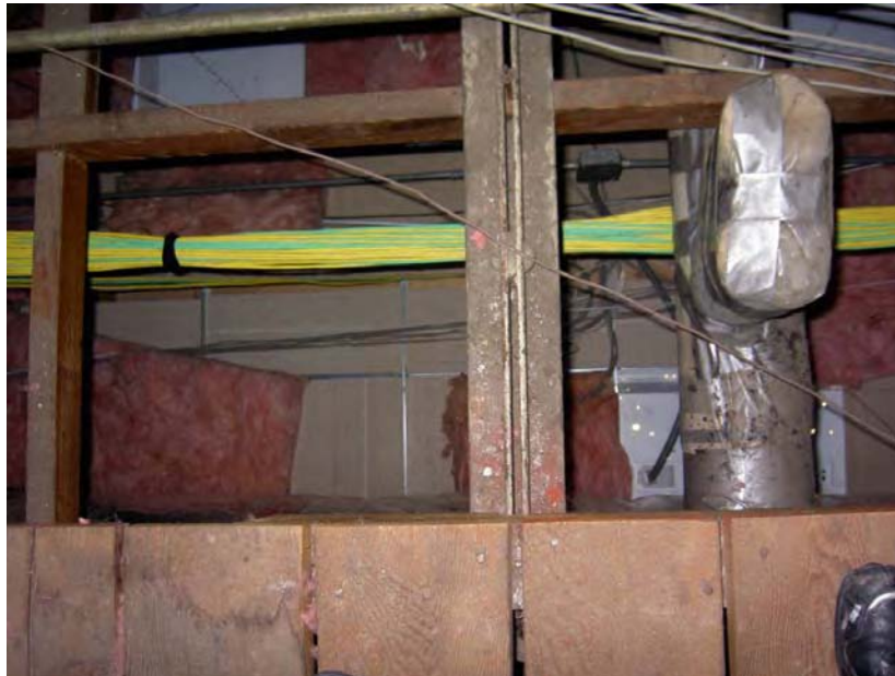
Figure 12. Improperly installed insulation above the false ceiling of Building 622 is very effective.
