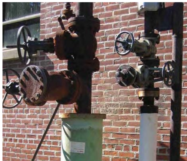
Figure 14. Uninsulated valves.
