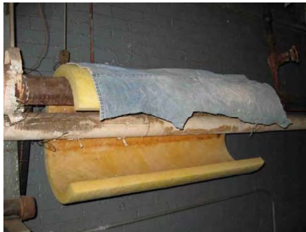
Figure 13. Uninsulated pipeline.
