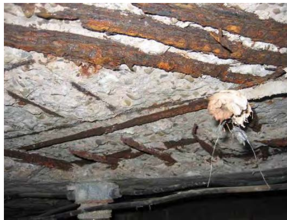
Figure 26. Closeup view of badly deteriorated condition of DH tunnels in the central steam distribution system.
