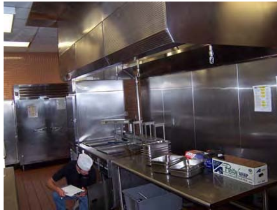
Figure 33. Typical kitchen hood with no extensions down or end skirts.
