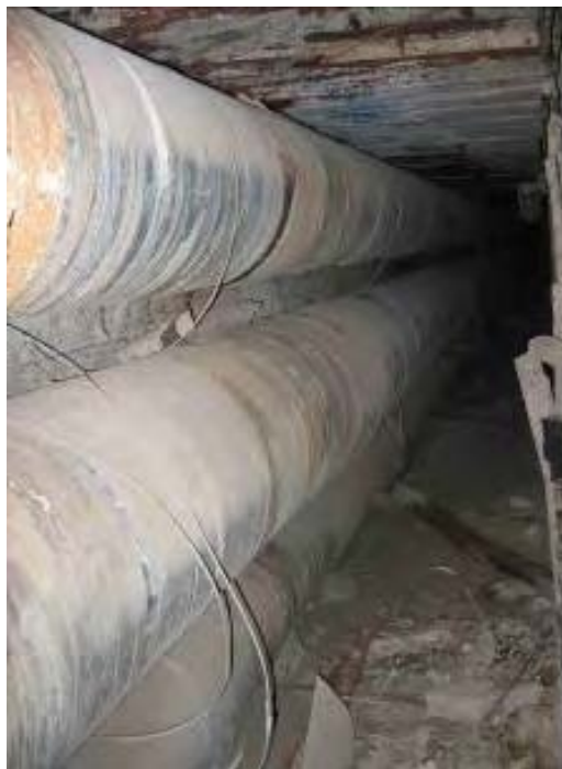
Figure 24. Pipeline systems in the central steam net and deteriorated condition of DH tunnels in the central system.
