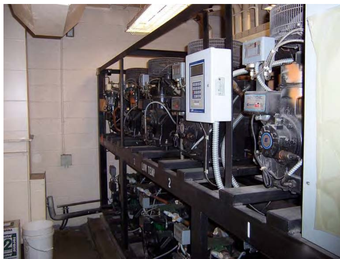
Figure 35. Rack of refrigerated room compressors.
