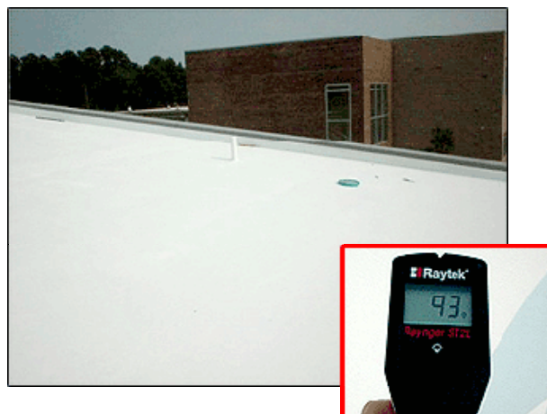
Figure 5. Dramatic decrease in roof air temperature after cool roof was installed.
