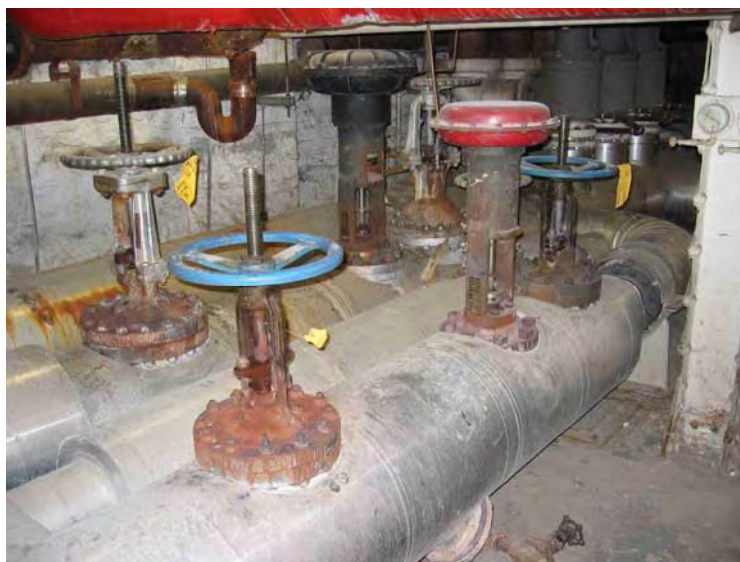
Figure 19. Pressure reducing valves in CEP 604.
