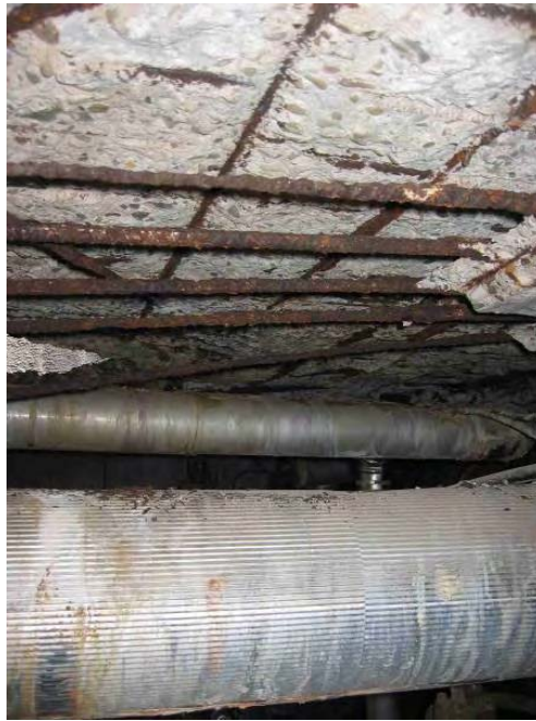
Figure 25. View of seriously deteriorated ceiling above central steam piping in DH tunnel.
