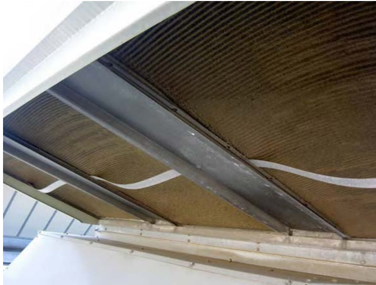
Figure 31. Filters in rooftop air handlers not properly maintained.
