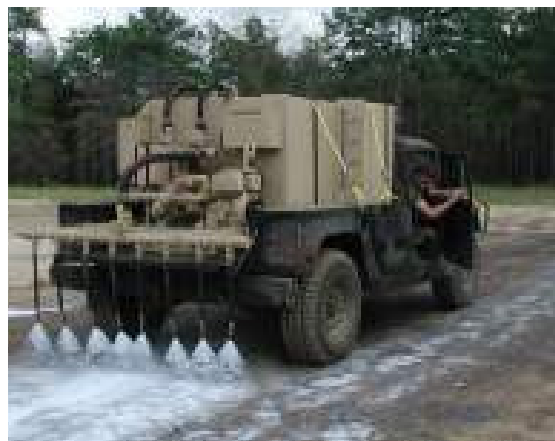
Figure 2-3. A sprayer equipped HUMVEE spraying emulsion polymers over the soil. (Newman 2005)
