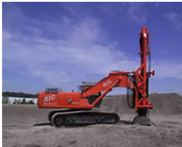
Figure 7-3. RIC (2004) compacting soil.
