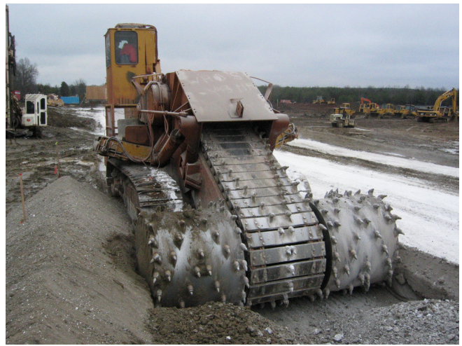
Figure 7-2. J. H. Becker Company equipment mixing lime into soil. (J. H. Becker, personal communication, 2005)
