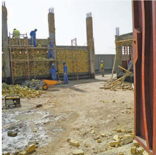
Construction work at the Basrah Modern Slaughterhouse.
