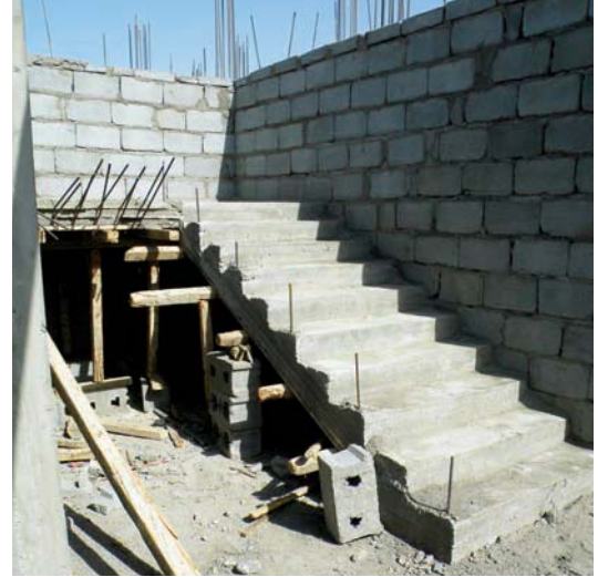
Construction of the Al Hadi Permanent Police Station.
