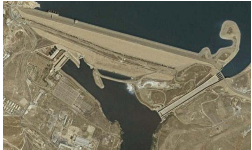
With higher water levels in the Tigris River, production of electric power at Mosul Dam increased to 419 MW this quarter, up 93% from last quarter. (Photo copyright GoogleEarth and DigitalGlobe)
