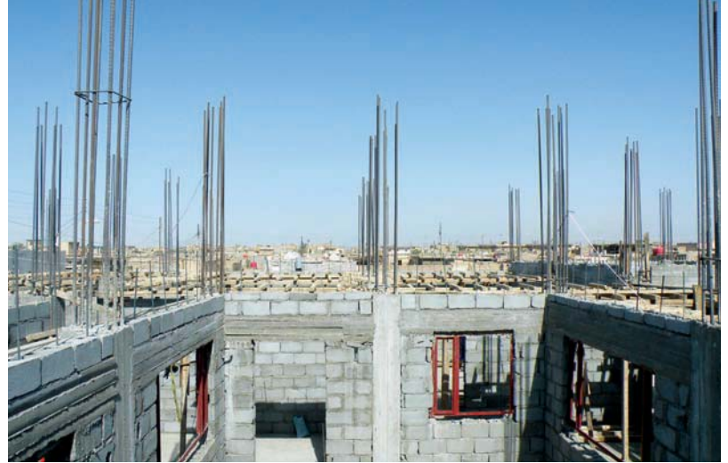
Construction of the Al Hadi Permanent Police Station.
