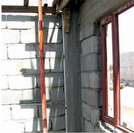
Expansion joint between infill and frame at Al Hadi Permanent Police Station.
