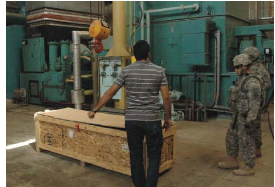
USACE personnel inspect one of two Rolls-Royce turbines at the Kharkh Water Treatment Plant. (USACE photo)
