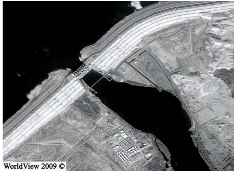
Aerial Imagery taken on December 10, 2009, of the Haditha Dam. (PA-09-192)
