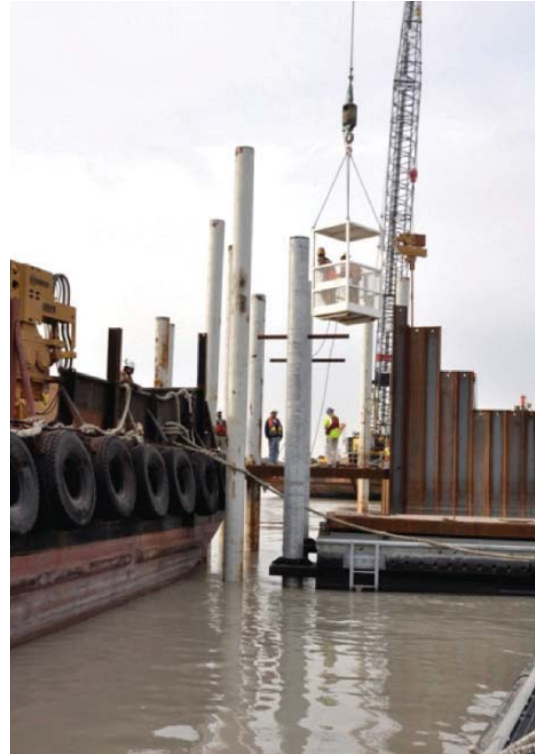
Construction of the $53 million pier and seawall continued this quarter at Umm Qasr in Basrah province. (USACE photo)
