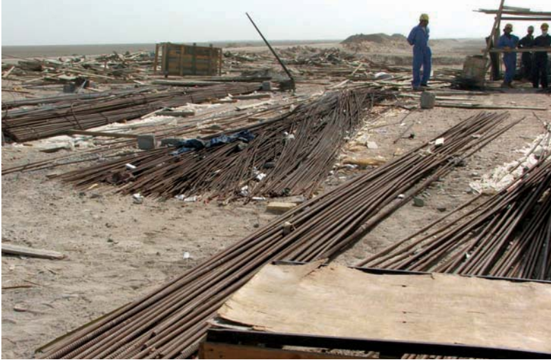
Reinforcing materials for the Basrah Modern Slaughterhouse.
