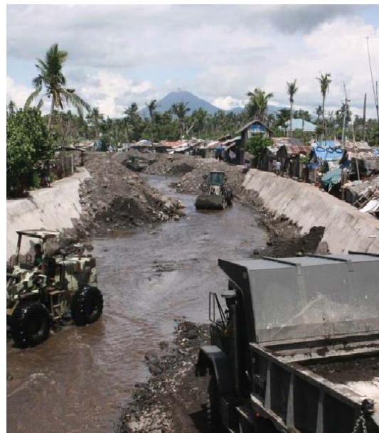
Doing construction work to improve local conditions.
