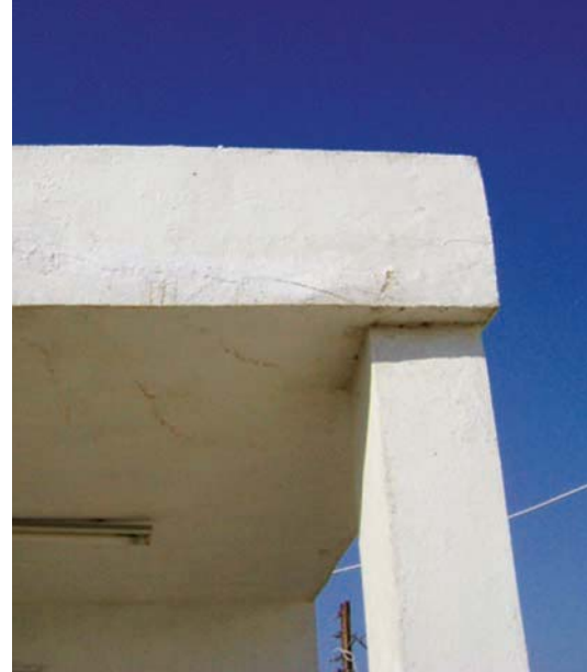
Contractor's "fix" for the reinforcement beam crack: stuff the crack with gypsum and paint over it. (GRC photo)
