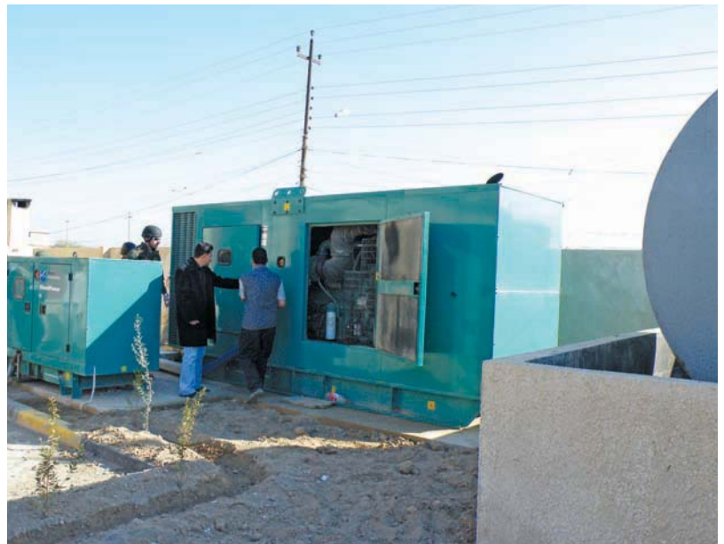
Two generators providing primary and emergency backup power for the Hai Tiseen PHC.
