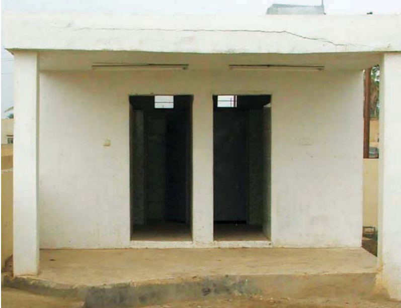
New latrine building with significant shear crack.
