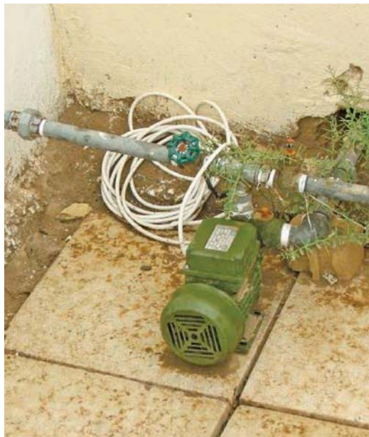
Exposed electrical wiring to the supply pump at the Khandek Intermediate School.
