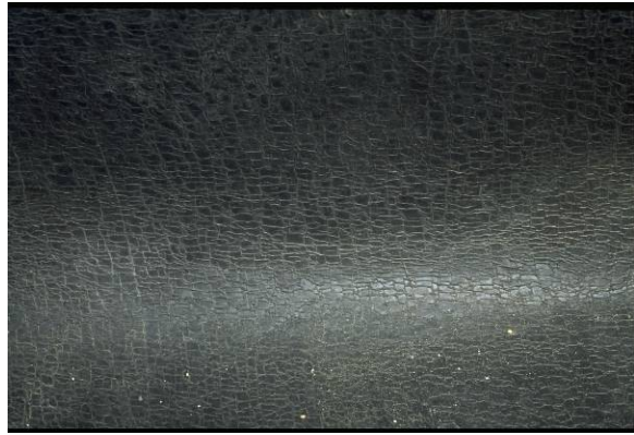
SR-L-3: On smooth liquid applied surfacing, there is evidence of crazing of top surface with hairline cracks (alligatoring).
