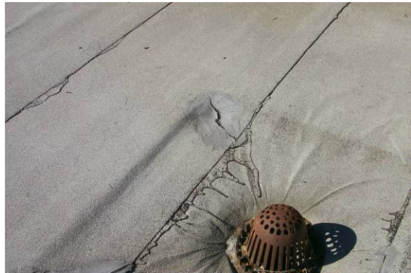
DR-H-1: Holes, splits, or tears in stripping ply caused by deterioration or physical damage.
