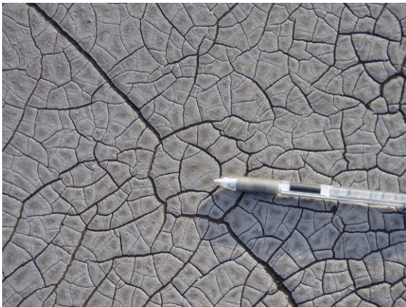
SR-M-4: On smooth liquid-applied surfacing, alligator cracks extend down through coating to the surfacing ply.
