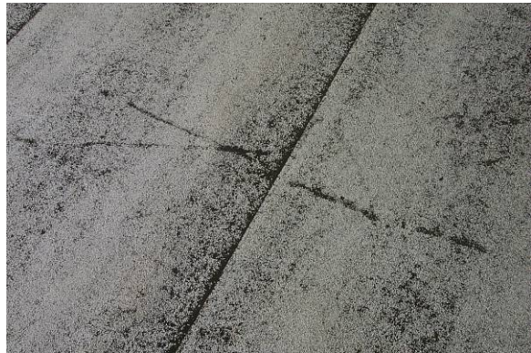
SR-M-2: On mineral surfaced capsheet surfacing, there is loss of granules, exposing the surfacing ply.
