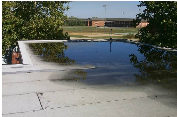
PD-L-1: Ponding is rated low severity due to the maintenance problems associated with it.
