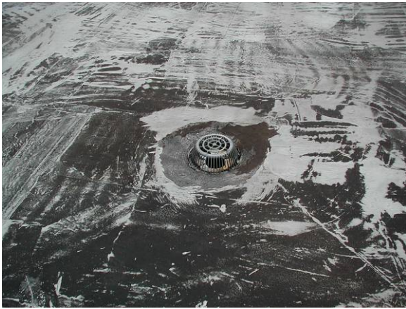
SR-L-2: On smooth liquid applied surfacing, there is loss of coating but no visible deterioration of surfacing ply.
