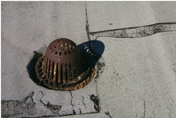
DR-M-4: Field seam exists under clamping ring.
