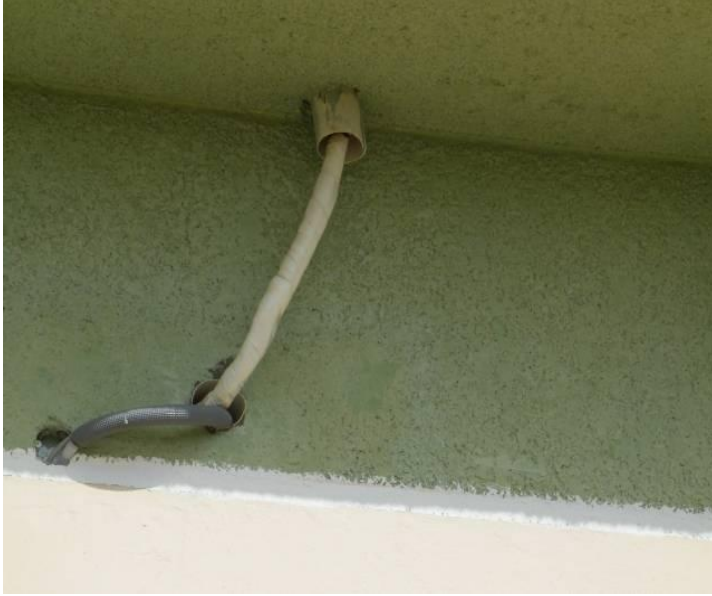
Site Photo 5. Coolant line penetrating roof and wall
