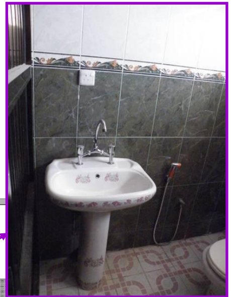
Site Photo 8. Restroom
