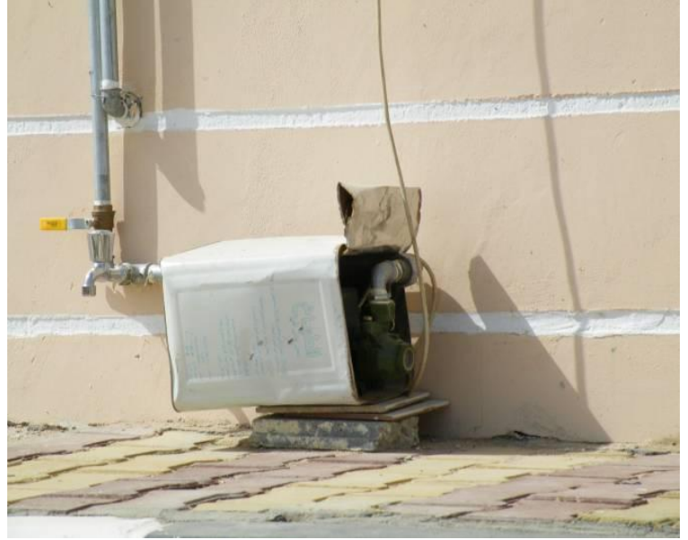
Site Photo 6. Water transfer pump
