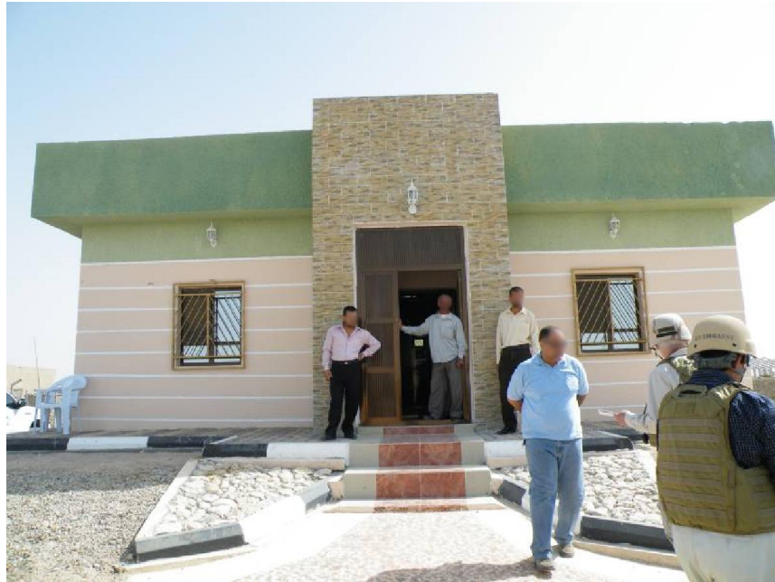
Site Photo 4. Building front exterior
