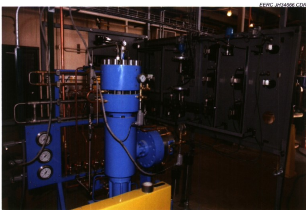
Figure 7. The gas compressor and the back of the board holding gas-blending valves and regulators.
