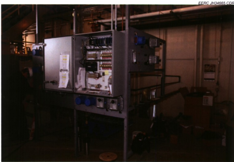
Figure 6. The air-purged electronics box in which all electronic connections are made.
