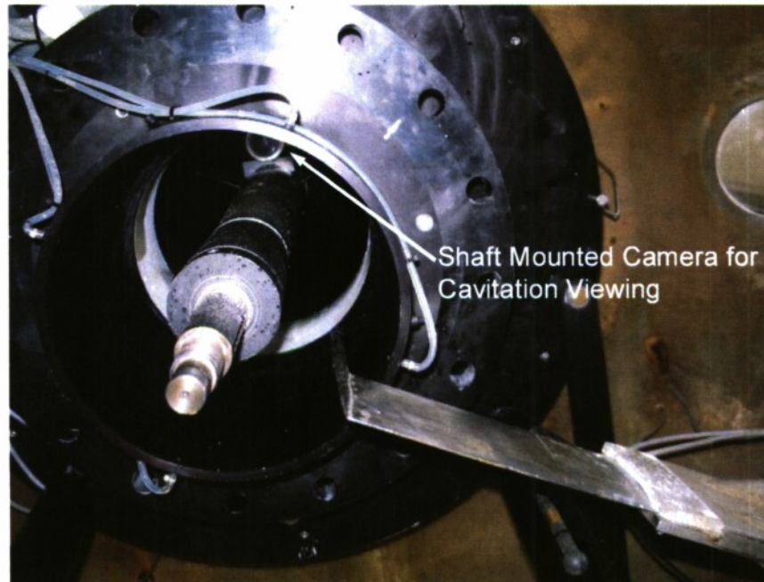
Fig. 7. Shaft camera mounted upstream of bellmouth in 36VPWT for cavitation viewing.
