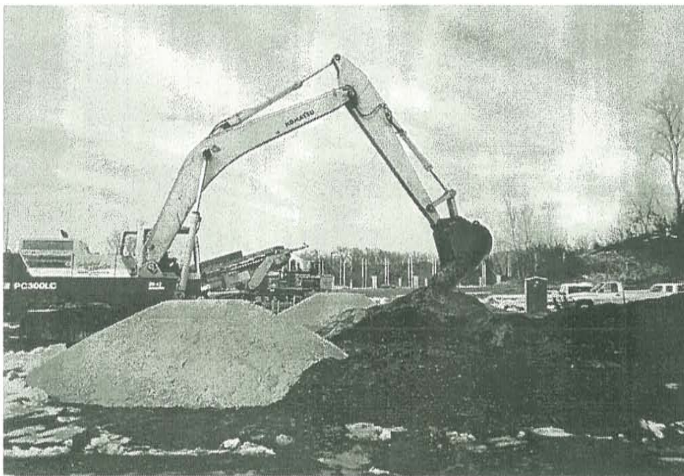
Figure 3a) Mixing of Mulch with Concrete Sand
