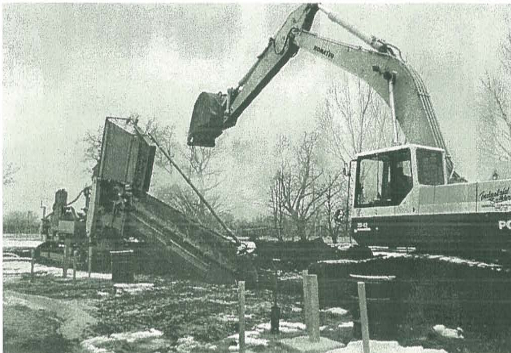
Figure 3b) Installation of the Biowall Using a Continuous Trencher
