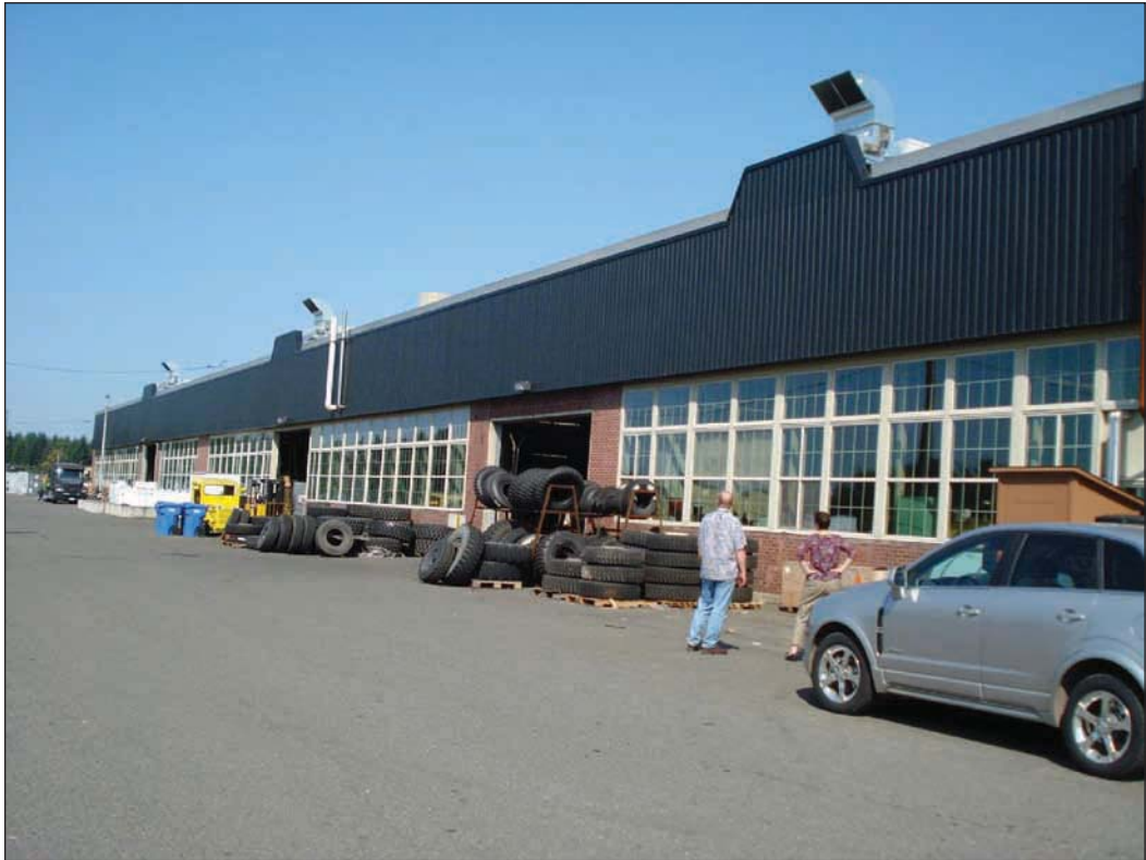
Figure 2.6 Fort Lewis Solar Wall on a Logistics Warehouse
