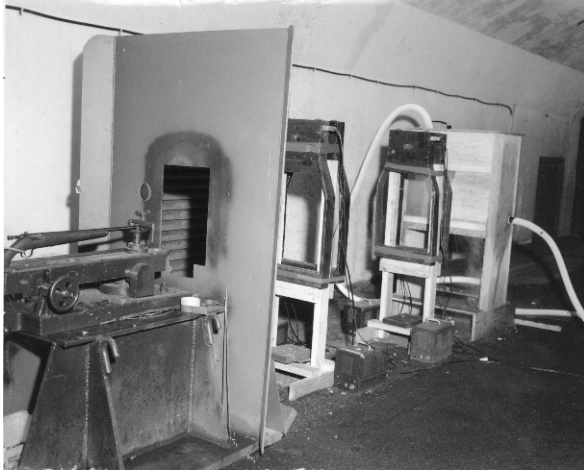
Figure 2. A plate being cooled with carbon dioxide before an armor acceptance test in 1962
