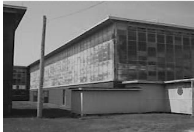
Priming Wing, Glass Pane Windows
