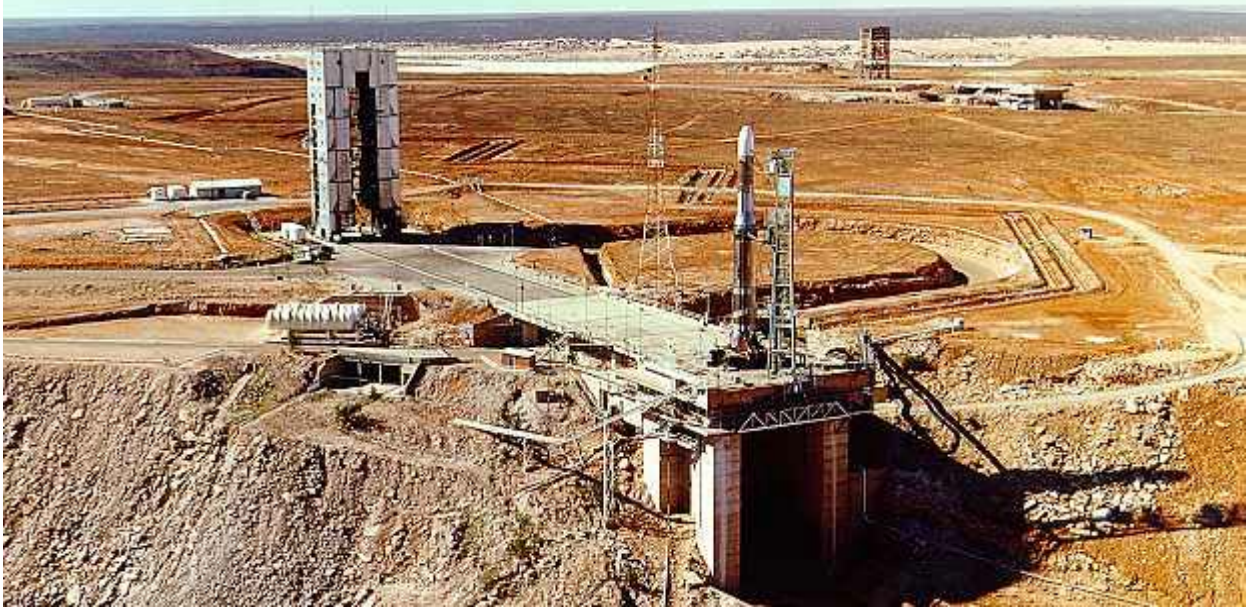
Figure 26. The ELDO launch site at Woomera with an Europa vehicle on the pad. The roll-away vehicle assembly building is the tall structure in the background. The paved access road goes in front the vehicle assembly building and circles under the concrete roll-out platform. Our preparation area, unfinished in this picture, was beneath the roll-out platform forward of the access road. The launch complex in the far background was dismantled and the dirt roads were overgrown by 1974. The image was taken from http://homepage.powerup.com.au/~woomera/eldo.htm .
