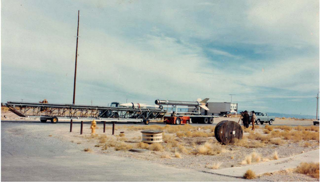
Figure 18. The HI STAR payload being mated to the Aerobee 170 before being mounted on the Nike booster in the tower. Note the plastic bagging around the payload for contamination control.
