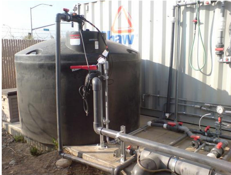
Figure 5.22 Spiking study plant effluent 20,000 gallon holding tanks.
