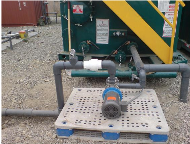
Figure 5.23 Spiking study recycle pump.
