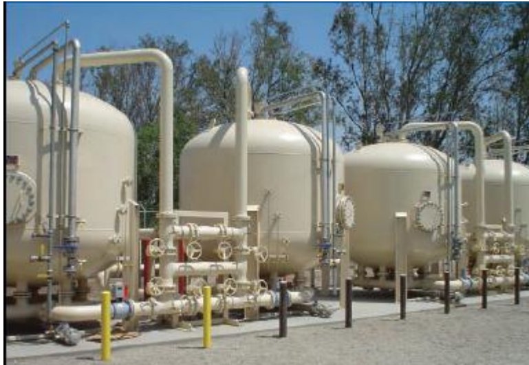
Figure 7.1 Typical ion exchange technology set-up with a lead/lag vessel configuration (Photo courtesy of Siemens Water Technologies Corporation).
