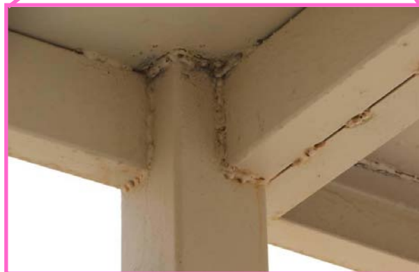
Site Photo 4. Poor weld quality at connections
