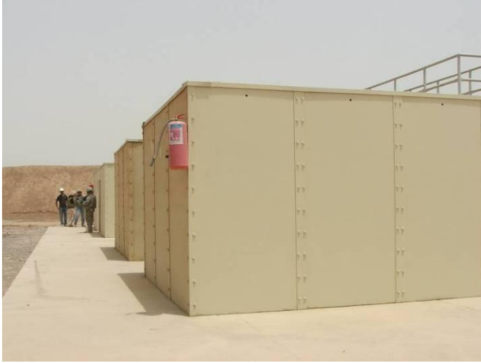
Site Photo 13. MOUT facility exterior
