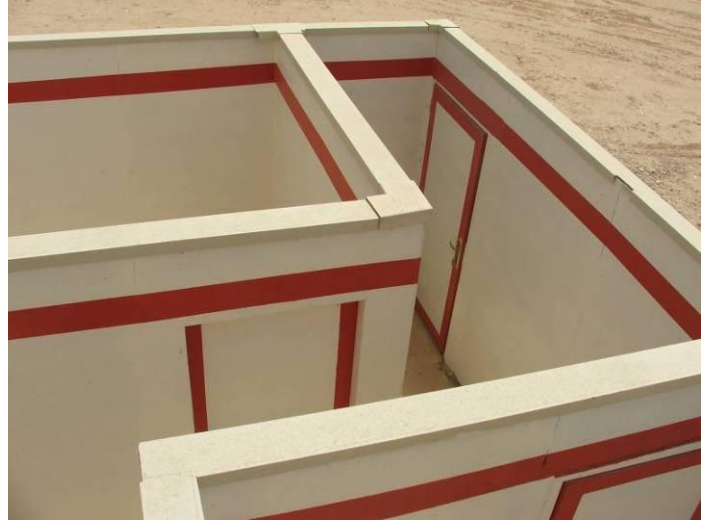
Site Photo 14. MOUT facility interior
