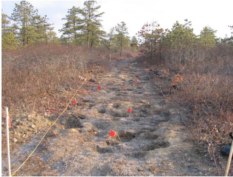
(a) Flags indicate subsurface anomalies along path being cleared for well pad
