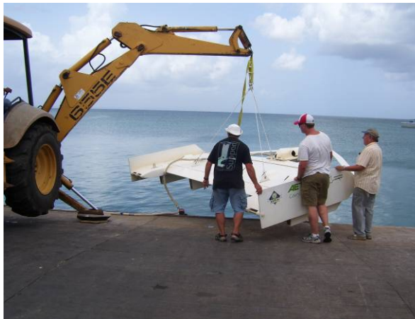
Figure 8-3. Because there was no boat launch facility, the MTA sensor platform is being launched from the Ferry Dock using a backhoe.
