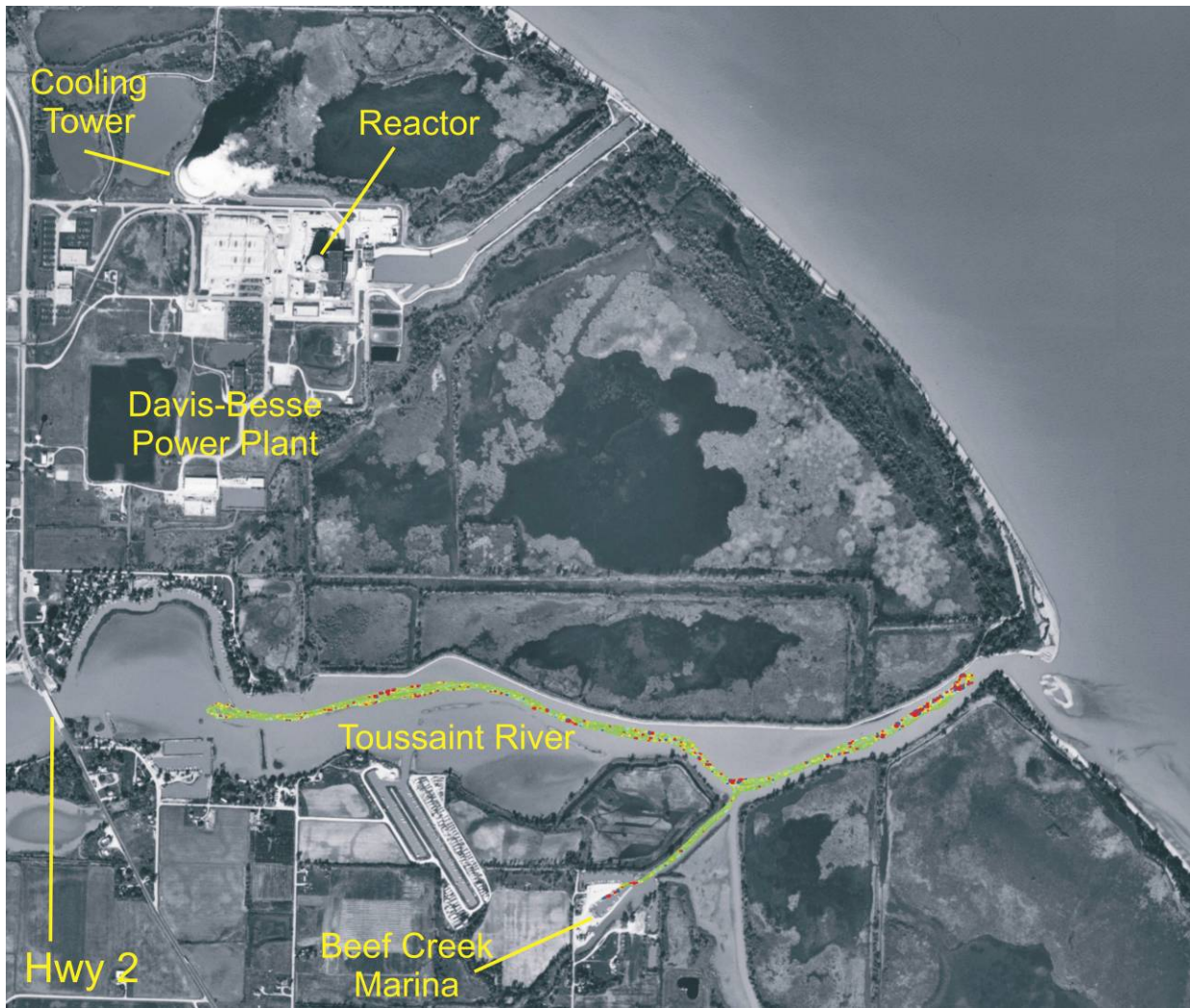
Figure 6-3. This 1996 aerial photograph shows the Toussaint River and the Davis Besse Power Plant. The magnetic anomaly image map of the MTA river survey is shown superimposed on the photograph.
