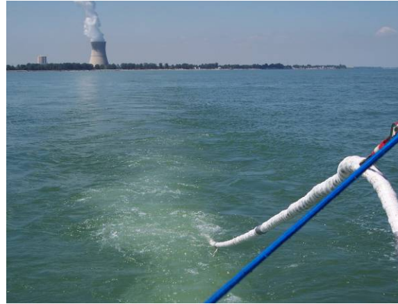
Figure 6-9. The MTA is shown surveying about 3 miles offshore from the Davis Besse Power Station.
