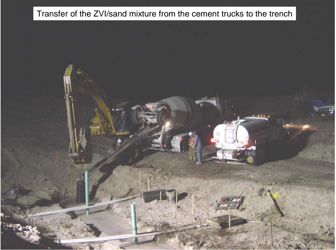
Transfer of the ZVI/sand mixture from the cement trucks to the trench
