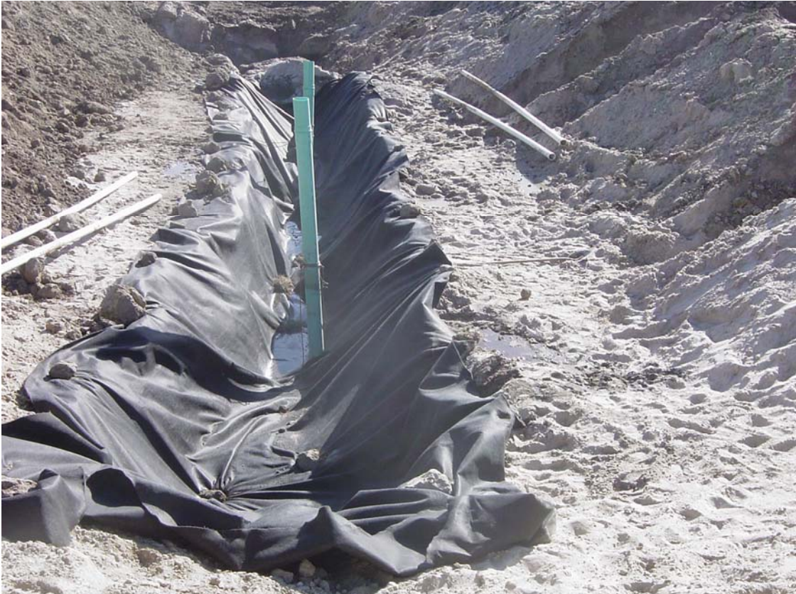
Geotextile placed in the top of the trench prior to clay addition
