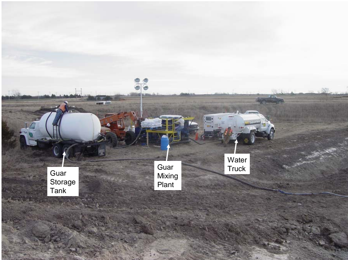
Removal of the overburden
