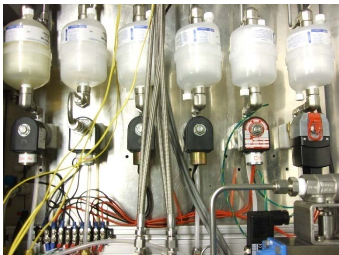
Figure D-3. Solenoid regulators
