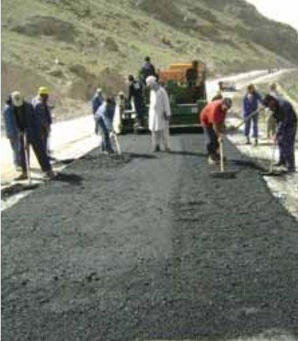
Placement of asphalt on the Mahmood Raqi to Nijrab Road. (Kapisa PRT photo)
