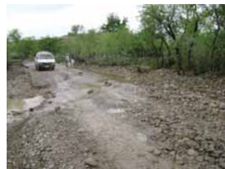
The Mahmood Raqi to Nijrab Road in Kapisa Province before construction. (Kapisa PRT photo)
