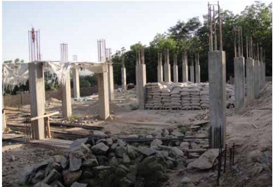
Unfinished work not removed from earlier construction at Habib Rahman Secondary School, causing major design and safety issues. (SIGAR photo)
