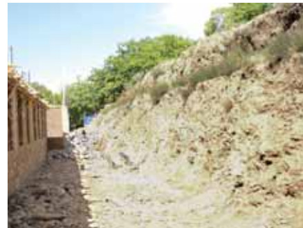
Back wall of Habib Rahman Secondary School showing the lack of a reinforced retaining wall, posing a hazard from potential rock and mudslides. (Kapisa PRT photo)
