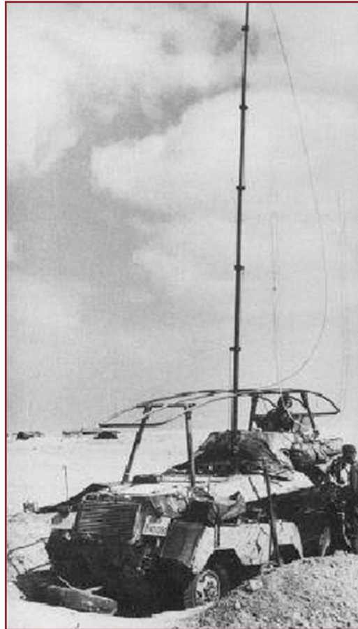
Fig. 2 Stryker-like Sd.Kfz-232 heavy armored wheeled command-post vehicle circa 1938. Note use of both the NVIS "frame" (horizontal loop) antenna for long-distance wide area on-the-move communications reflected off the ionosphere and a long efficient vertical monopole antenna for shorter distance "ground wave/surface wave" LOS communications. Facility communications were self-contained and capable of on OTM operation. NVIS was the primary mode of OTM omni-directional communications. A short vertical (whip) antenna was also provided for short distance OTM LOS communications.
