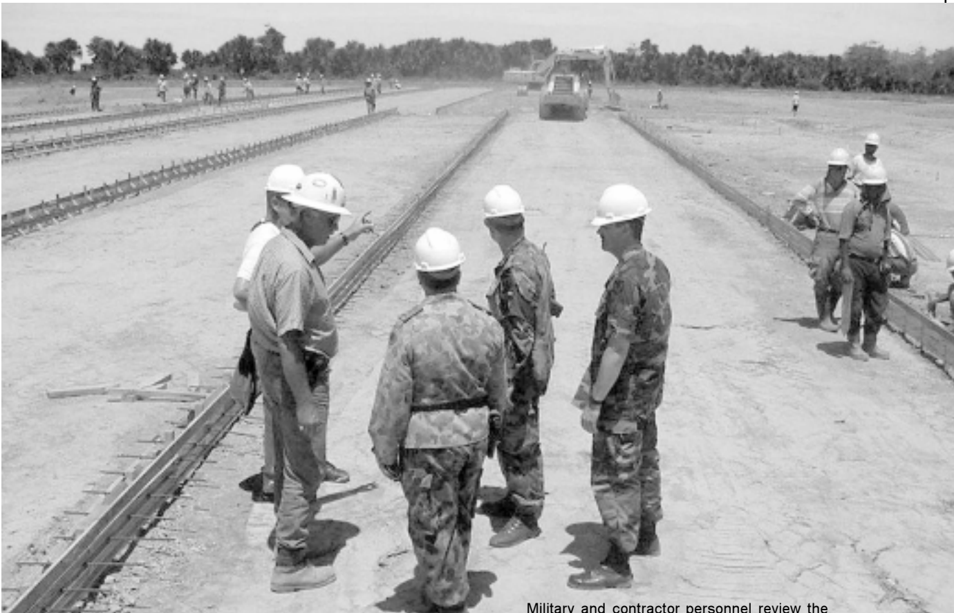
Military and contractor personnel review the construction of helicopter pads at East Timor's Dili Airport. (Inset) A contract Mi-26 helicopter and C-130 Hercules parked at the airport.
