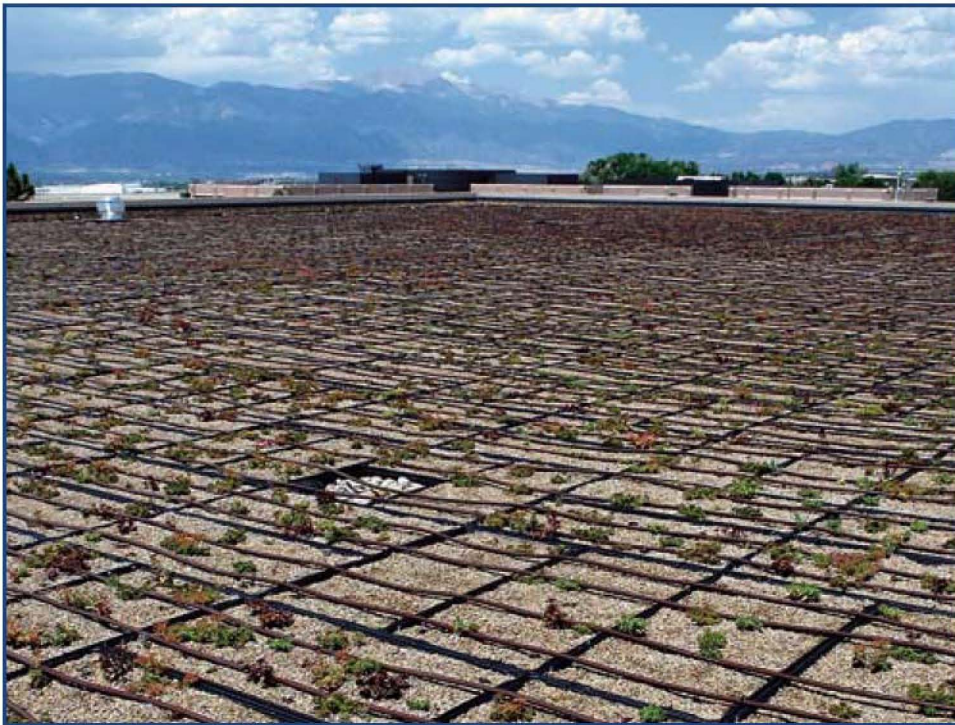
Vegetative roofs can help cut down on utility bills as well as rainwater runoff by insulating the roof from the heat of the sun and capturing the rainwater for the plants. The Air Force is testing the concept on an administrative building at Peterson AFB.
