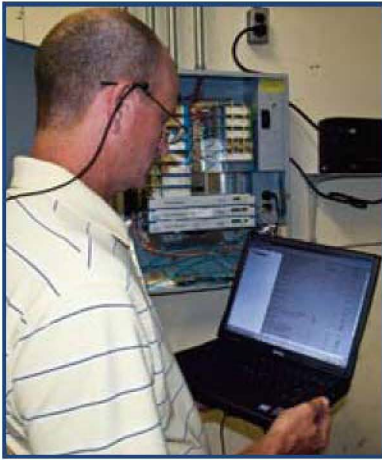
An Energy Management Control System (EMCS) technician at Tyndall AFB configures a Direct Digital Control (DDC) panel to communicate with the EMCS central server. EMCS operators monitor and control building HVAC systems from the server front end.
