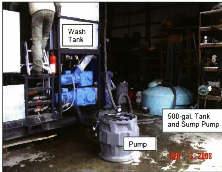
Figure 6. Material Rinsing Water Routed off the Main System through an Intermediate Sump Pump and into a 500 Gal Tank
