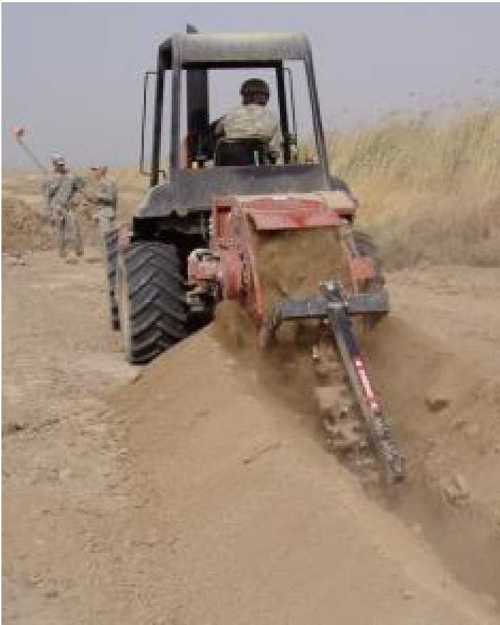
Soldiers digging a trench for fiber optic cable at Contingency Operating Base Speicher, Iraq.
