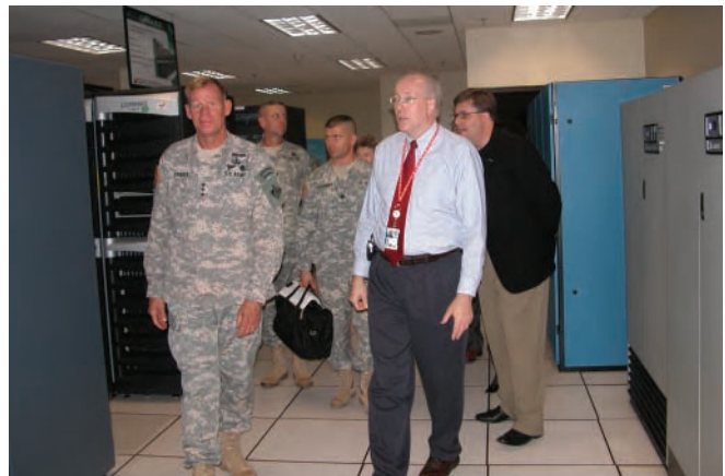
LTG Carl A. Strock (far left) walks through Joint Computing Facility as Dr. Jeffery P. Holland (second from right), ERDC Acting Deputy Director, and John West (far right) discuss supercomputing infrastructure, July 18
