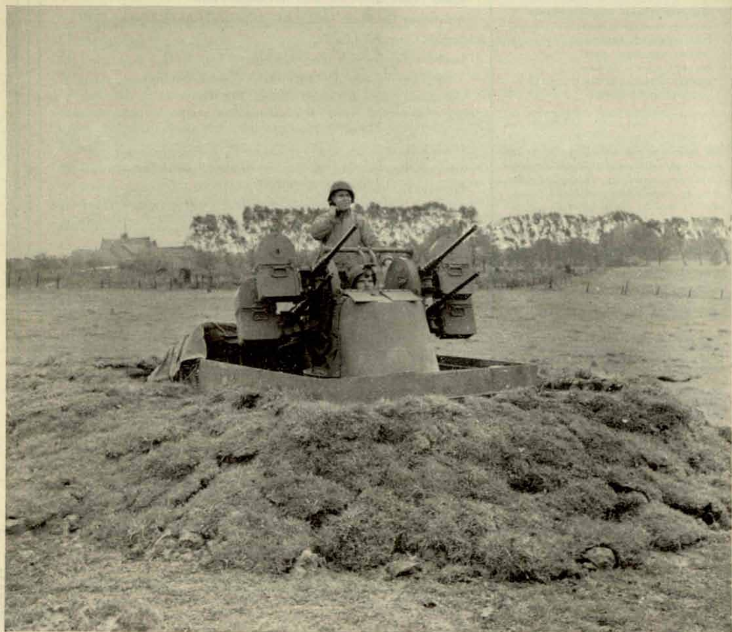
Using sod camouflage, Battery C, 554th AAA AW Battalion completely dug in its M-15 Half Tracks.
